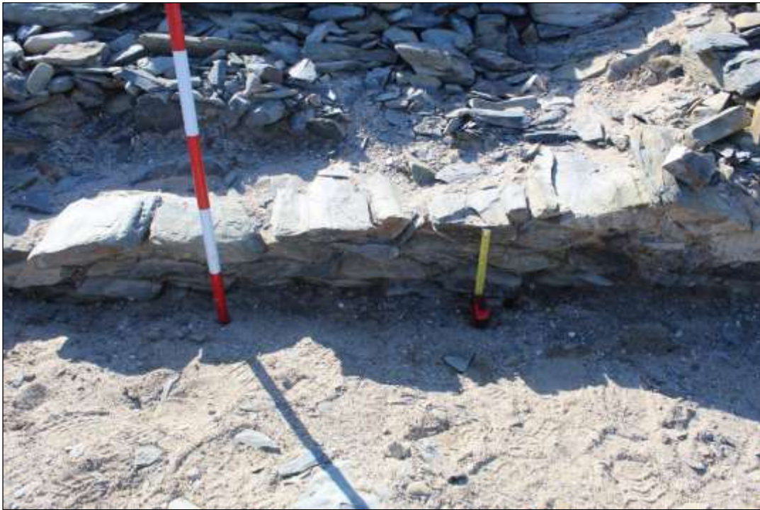
Figure 5: Foundation courses in the collapsed section of the BSQW exposed before the construction of the experimental wall. The longer side of the foundation stones are laid transverse to the course of the wall.
