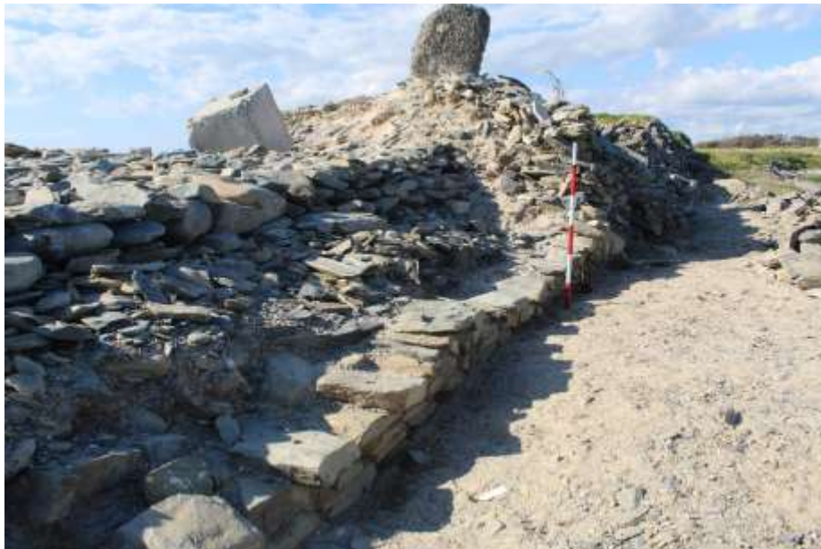
Figure 4: Foundation courses of the wall. View north shows a standing section of the wall with a sand deposit in the core of wall below a concrete cube.
