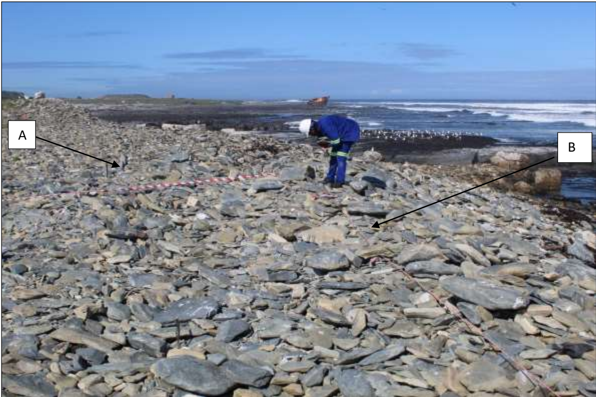
Figure 1: Two tie ropes, A & B, were laid parallel to each other along the collapsed section of the BSQW. They were used to guide the search for the foundation of the wall. Foundation courses were found 30cm to right of cord A.
