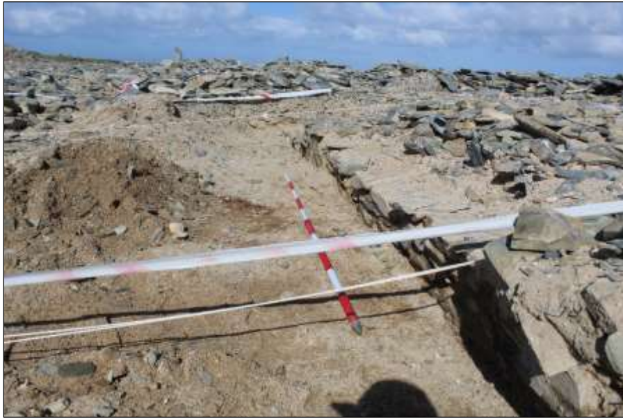
Figure 3. Foundation courses, view from the north.
