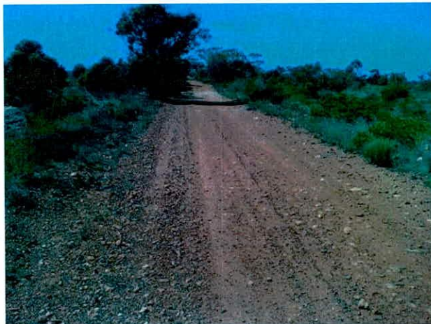
Figure 30: Gravel Access Road
