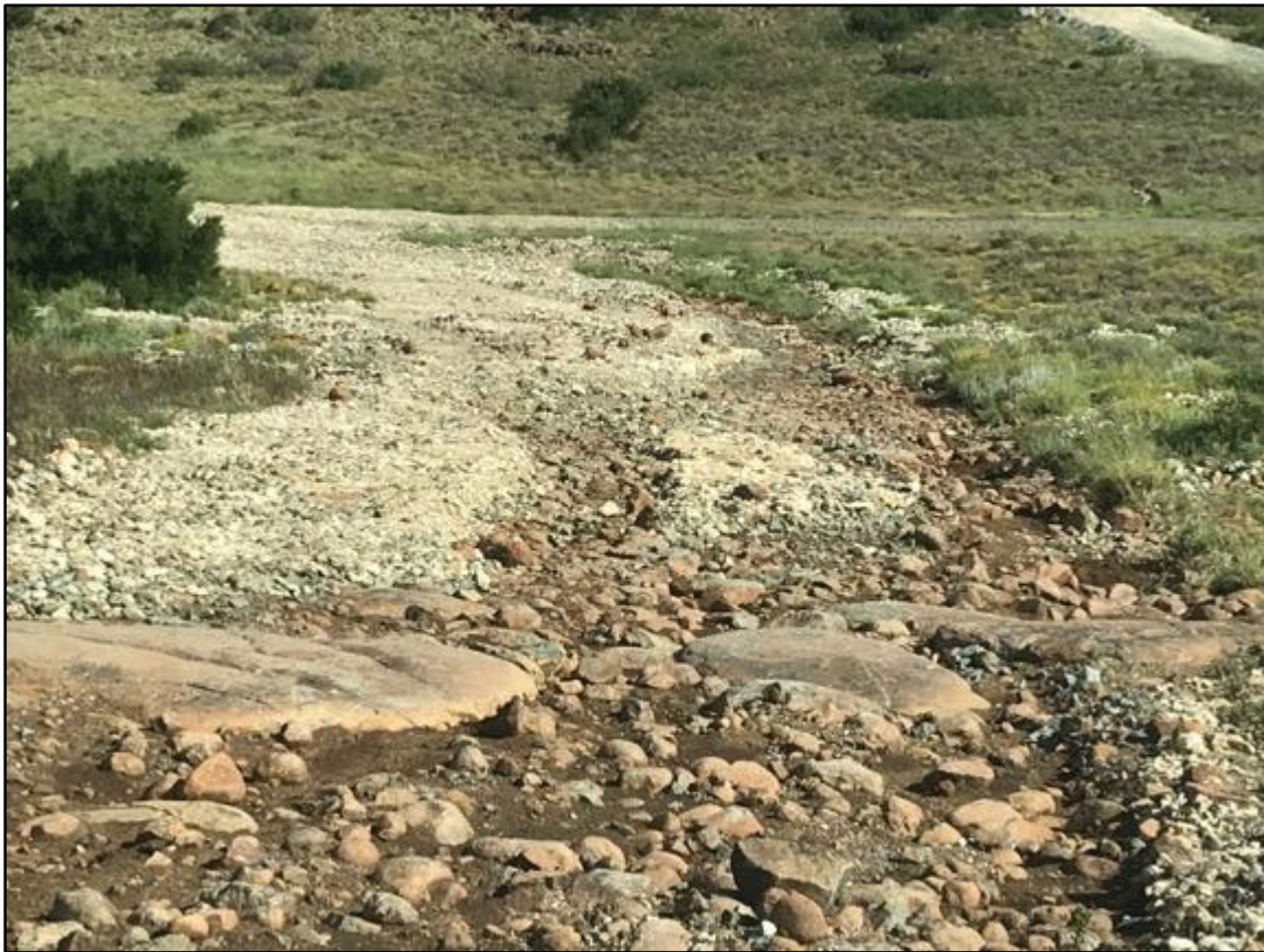
Figure 6: Example of perpetual erosion on steeply sloping gravel road.
