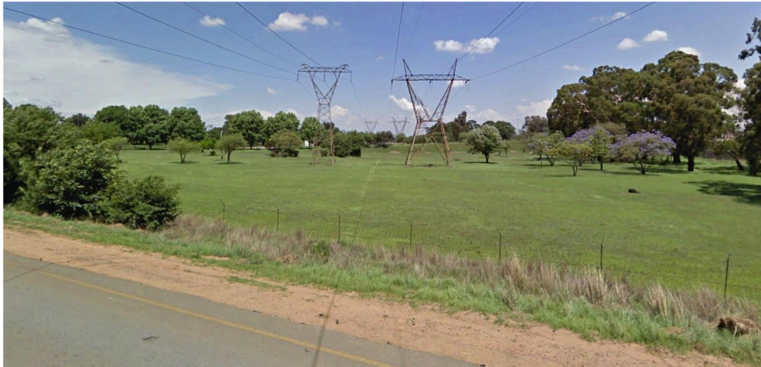
Figure 8: Grassland with low Visual Absorption Capacity (VAC) along a power line servitude compared to the high VAC of planted trees adjacent to the servitude.
