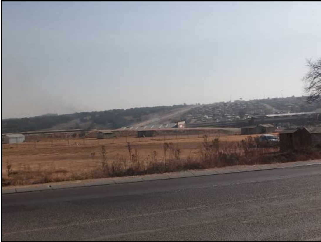
Photograph 3.2: Residential areas to the north of N4
