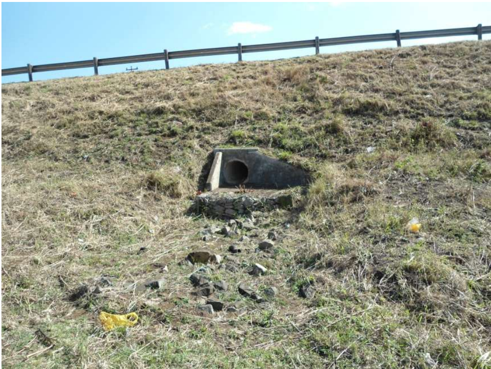
Plate 6: Culvert beneath N2, associated with Watercourse 3 (GPS coordinates: -28.411020°; 32.168393°)
