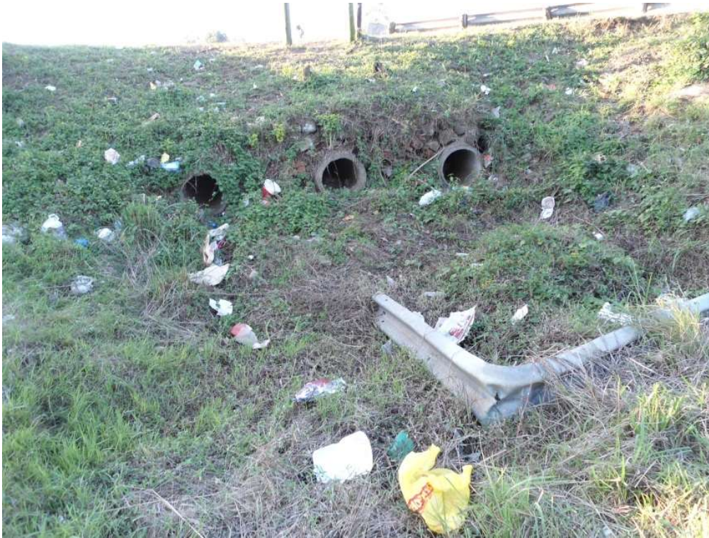
Plate 17: Culverts located beneath the unpaved road, associated with Watercourse 7 (GPS coordinates: -28.409735°; 32.184087°)
