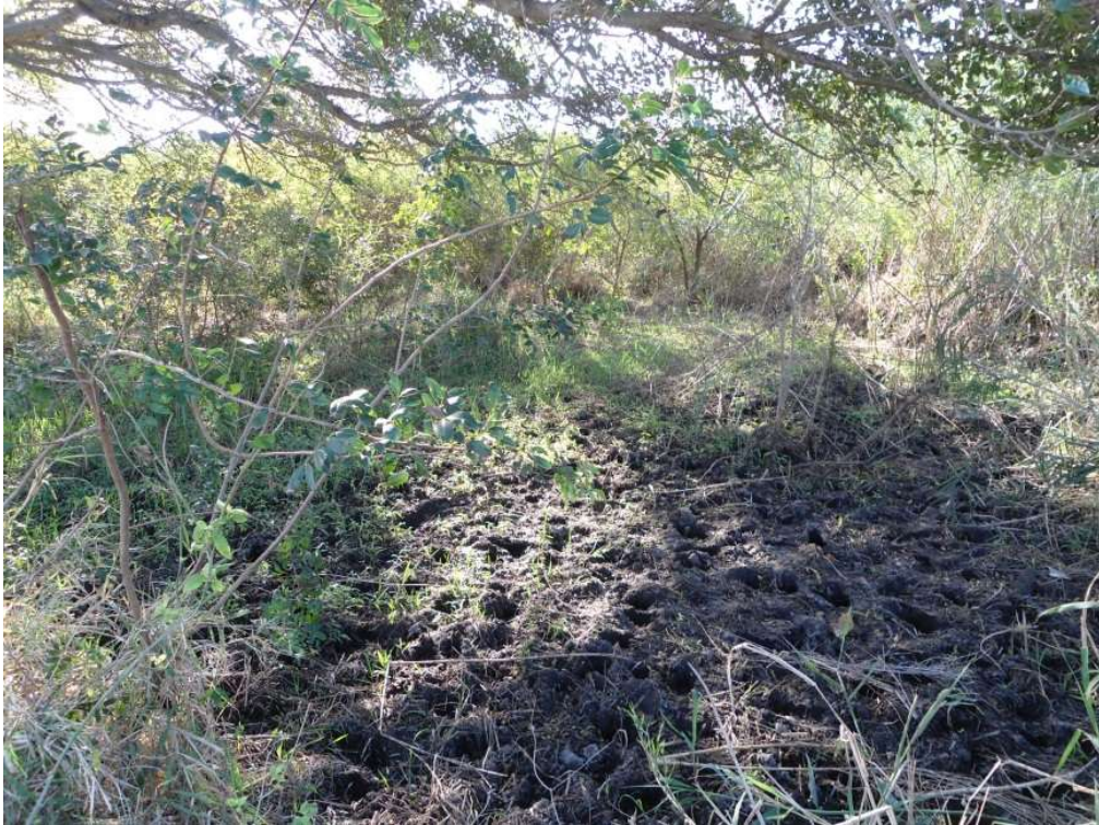
Plate 15: Dried watercourse in the vicinity of the access road culverts associated with Watercourse 6 (GPS coordinates: -28.408966°; 32.178130°)
