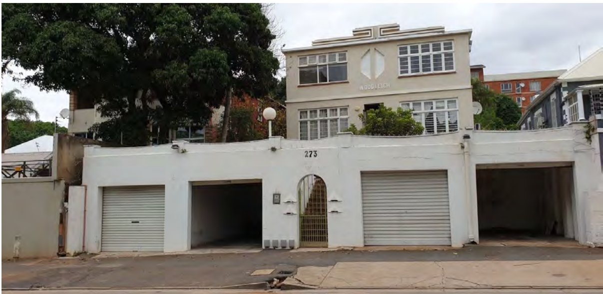
Figure 19 - Woodleigh flats at 273 Percy Osborn Road immediately adjacent and to the south of the application site.
