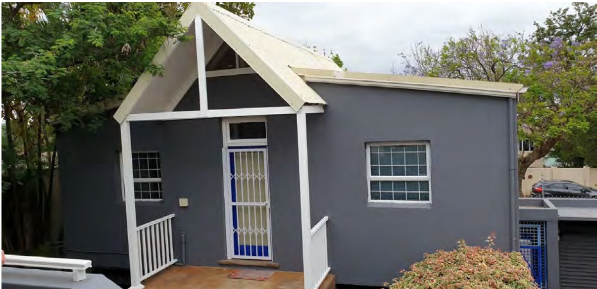
Figure 15 - View of existing primary outbuilding/ancillary unit from the steps of the house
