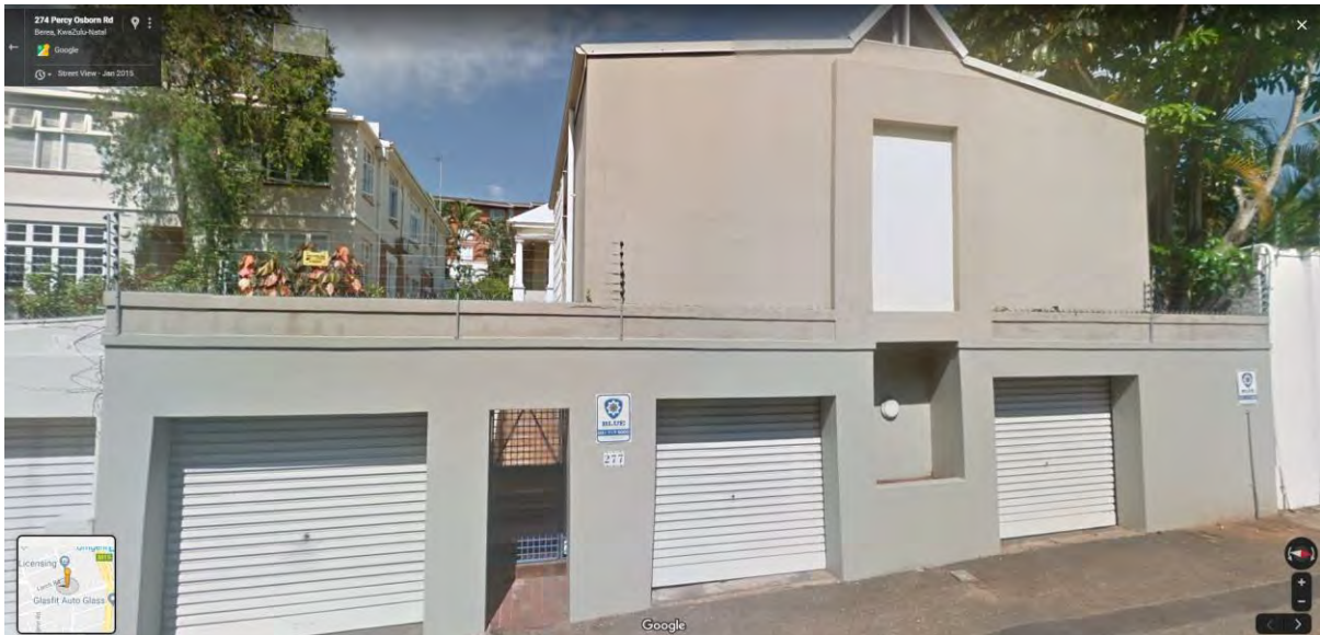
Figure 5 - Showing existing structures as viewed from Percy Osborn Road.
