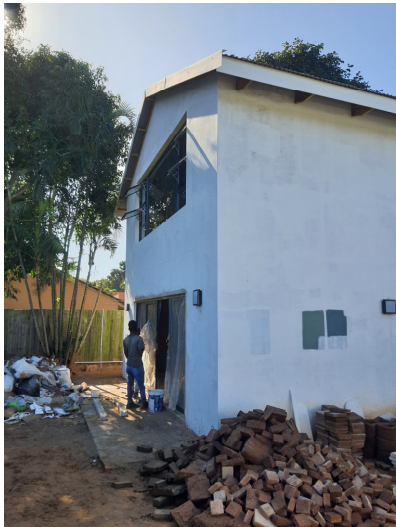
FROM THE RIGHT NW ELEVATION SHOWING THE DOUBLE STOREY ADDITION
