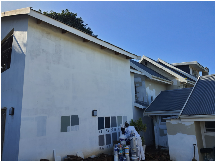
FROM THE LEFT SW ELEVATION SHOWING THE DOUBLE STOREY ADDITION
