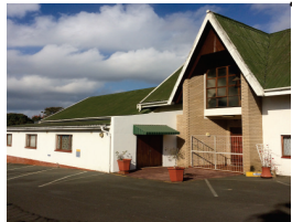
side elevation showing recent extensions to church building
