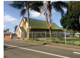
front facade and street view
