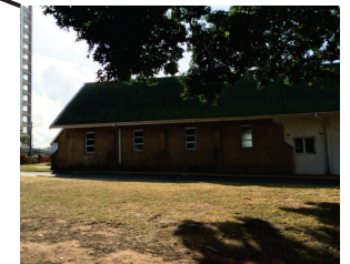
side elevation of existing church
