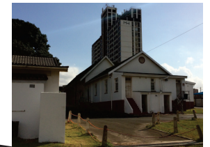
rear of existing dining hall & barrat house
