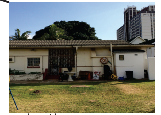
rear barrat house
