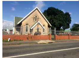
front facade and street view
