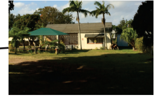
front facade barrat house
