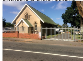
front facade and street view
