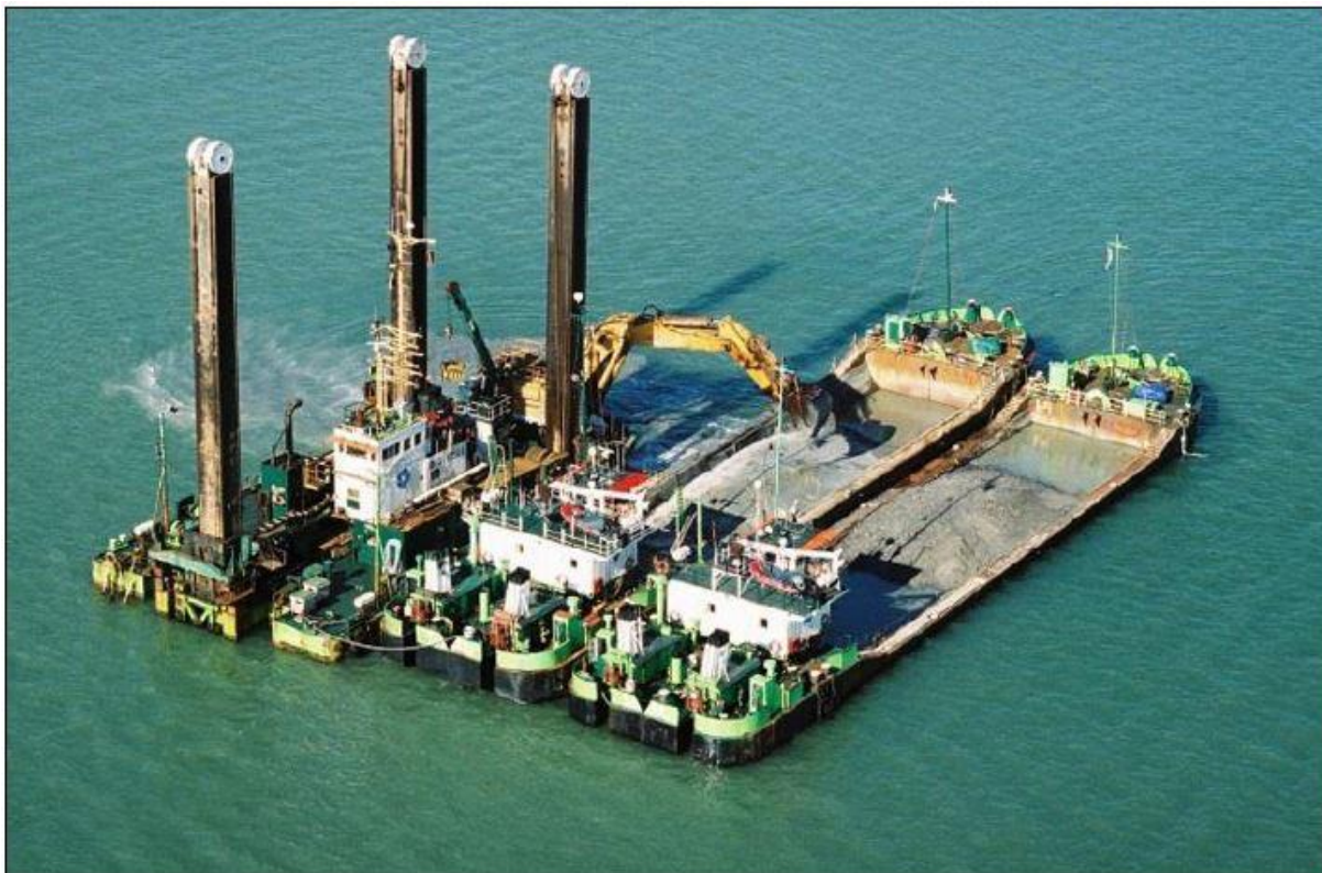
Figure 4: Backhoe dredger loading dredged material into self-propelled split barges (Source PRDW 2016).
