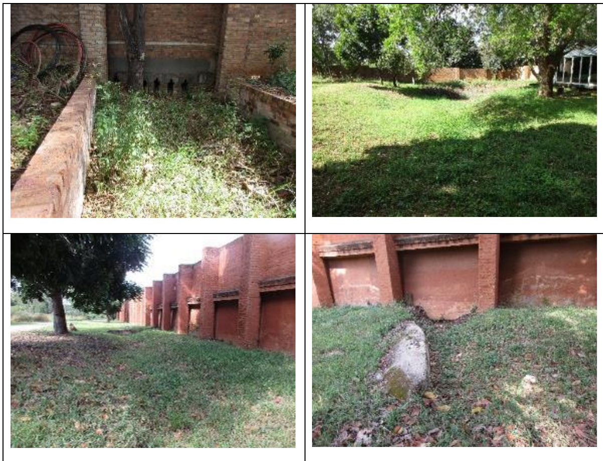
Figure 7.1: Images of the canal located on site.
