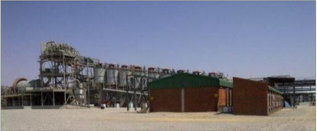
Figure 17: Existing Western Limb Tailings Retreatment facility showing flotation cells (middle) and ball mill (right). In the foreground is the proposed site for the four IsaMills™
