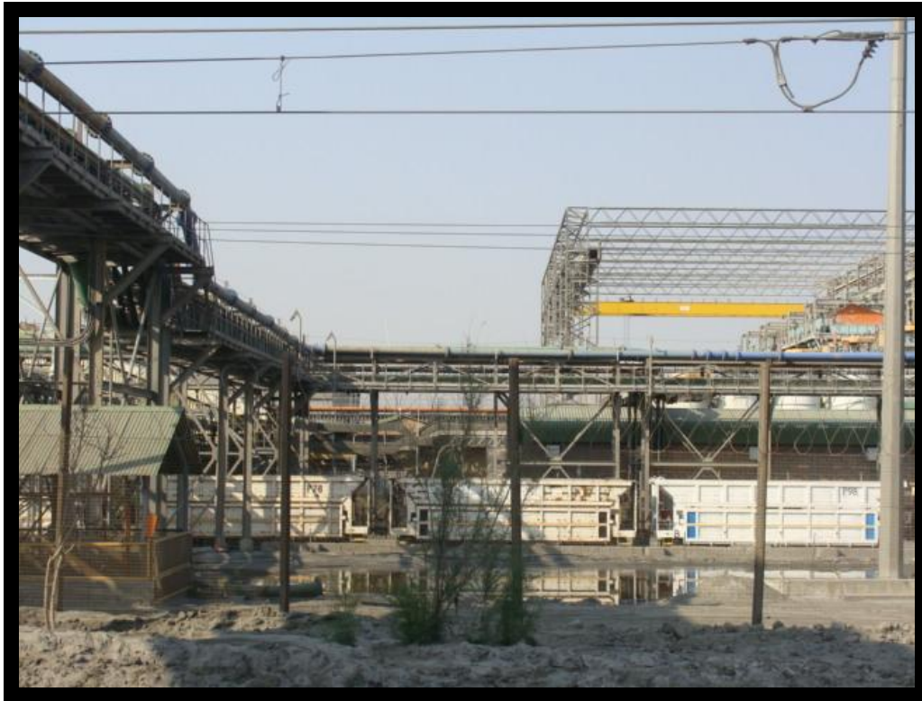
Figure 9: Infrastructure area where different piping will be placed.
