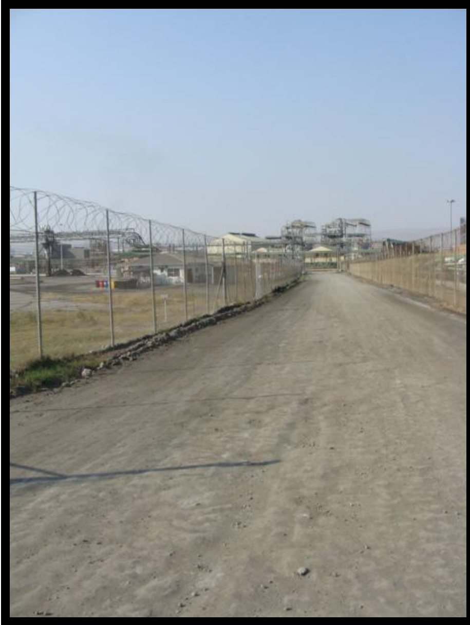
Figure 8: Area where the pump station is being proposed.
