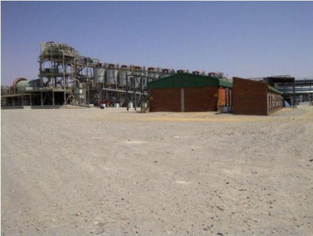
Figure 14: Existing Western Limb Tailings Retreatment facility showing flotation cells (middle) and ball mill (right). In the foreground is the proposed site for the four proposed IsaMills™
