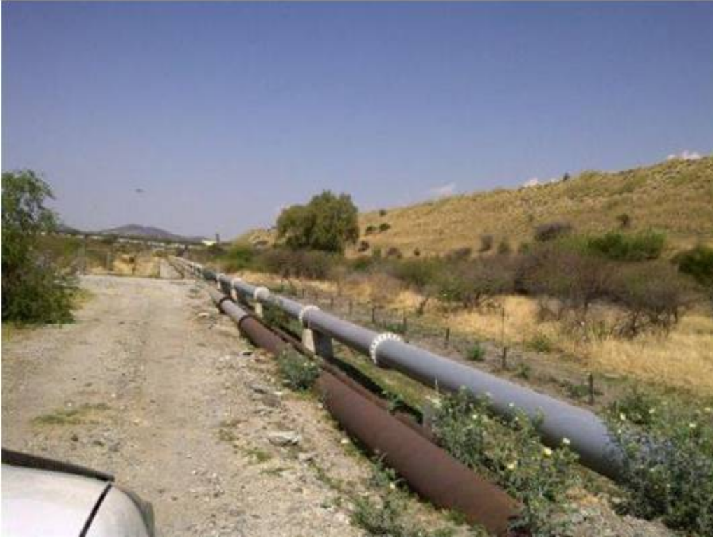
Figure 10: Example of overland pipeline
