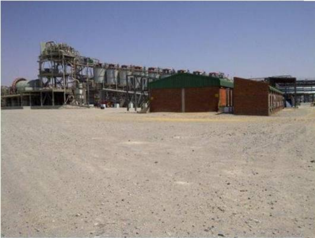
Figure 12: Existing Western Limb Tailings Retreatment facility showing flotation cells (middle) and ball mill (right). In the foreground is the proposed site for the four proposed Isa Mills™
