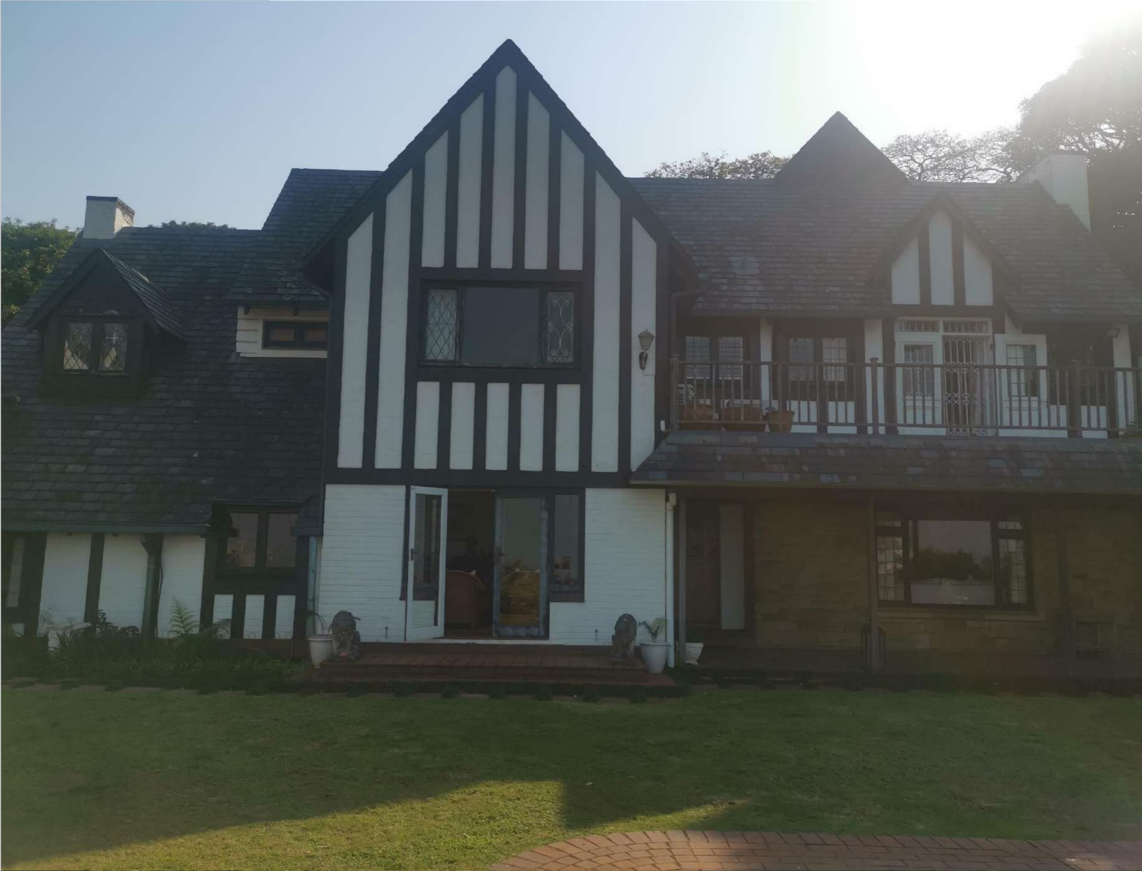
286 Innes Road Site Due Diligence | Amafa Demolition Application
