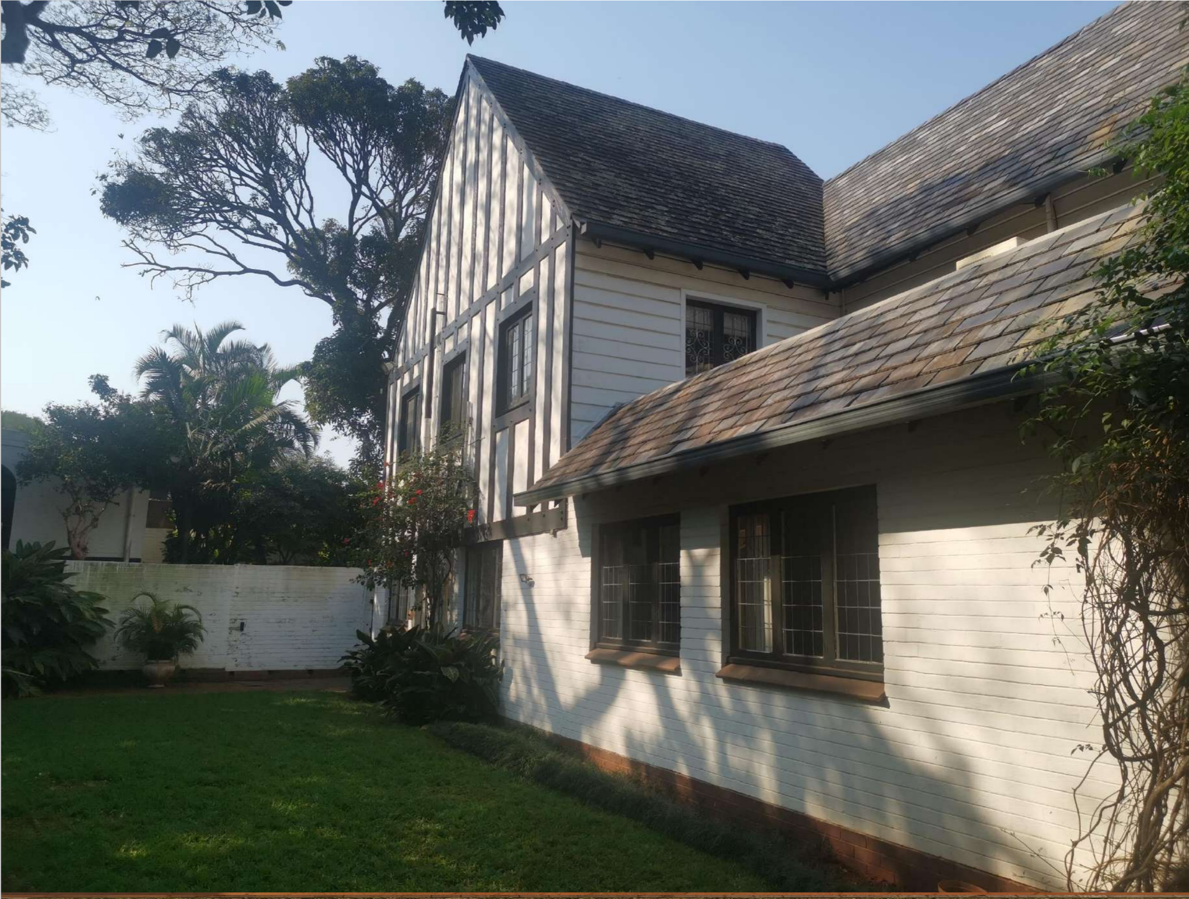
286 Innes Road Site Due Diligence | Amafa Demolition Application
