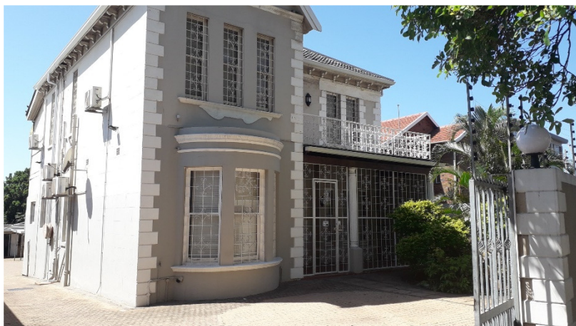
Fig. 8. View of 61 Bulwer Rd from inside the driveway gate
