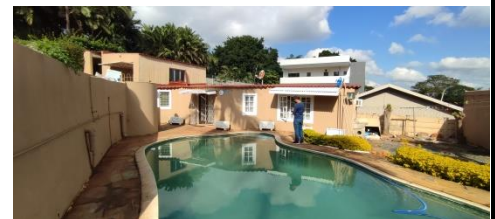
EXISTING OUTBUILDING AND GARAGE (NORTH FACADE)
