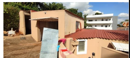
EXISTING OUTBUILDING AND GARAGE (NORTH FACADE)
