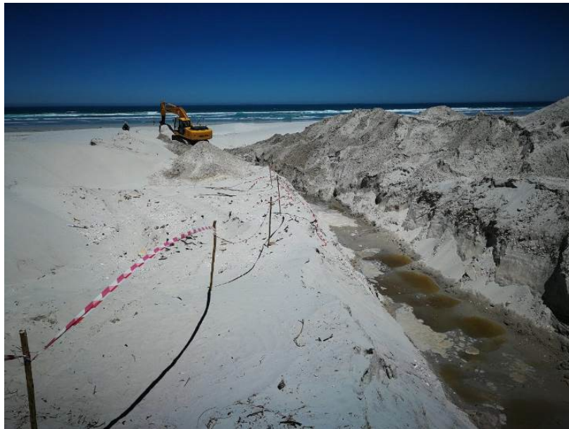
Figure 8 Example of excavations across the beach to bury the submarine cable
