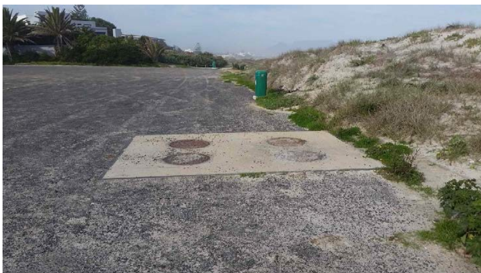
Figure 9 Example of an existing Beach Manhole
