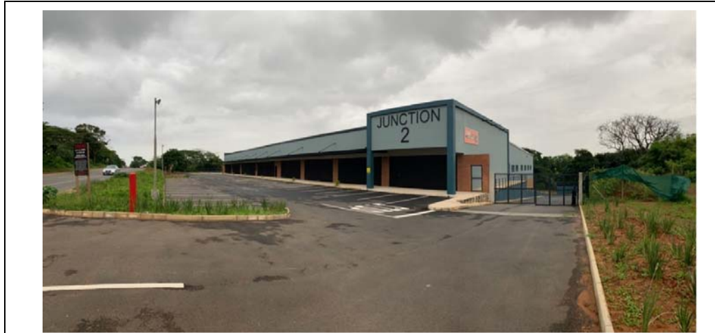
Plate 12 WIOCC's Cable Landing Station building at Umbogintwini
