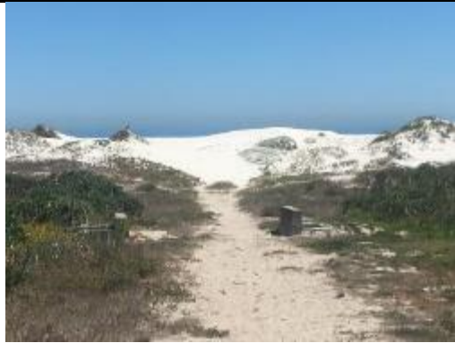
Beach access path under which the ACE cable sleeves have been installed. These will accommodate the 2AFRICA cable
