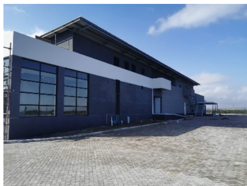
ACE Cable Landing Station under construction
