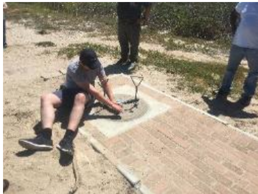
ACE BMH which will be used for the landing of the 2AFRICA/GERA (East) cable landing
