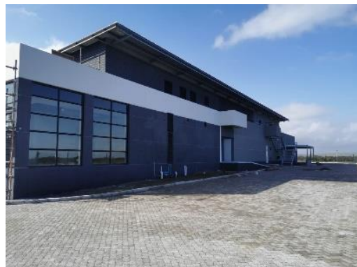
ACE Cable Landing Station under construction
