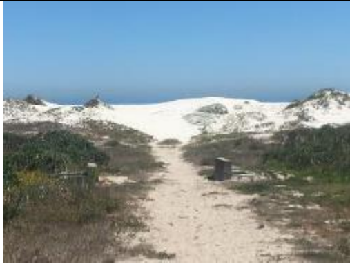
Beach access path under which the ACE cable sleeves have been installed. These will accommodate the 2AFRICA cable
