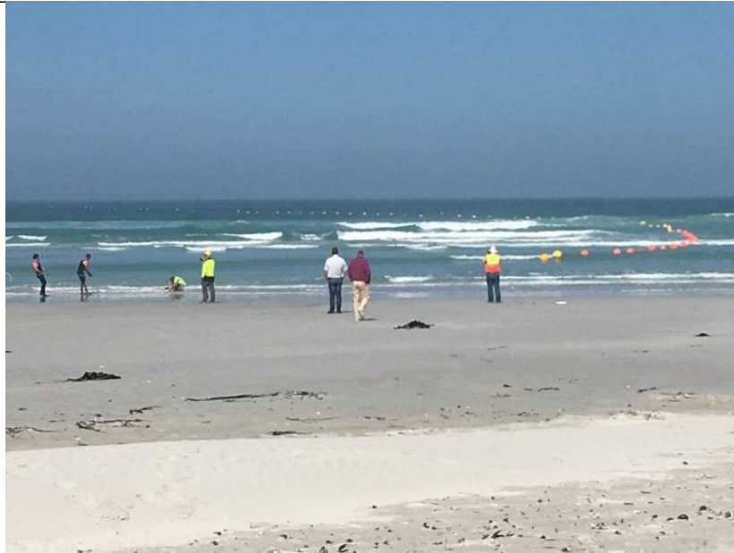
Figure 6 Example of a cable being guided to shore by divers and small boats
