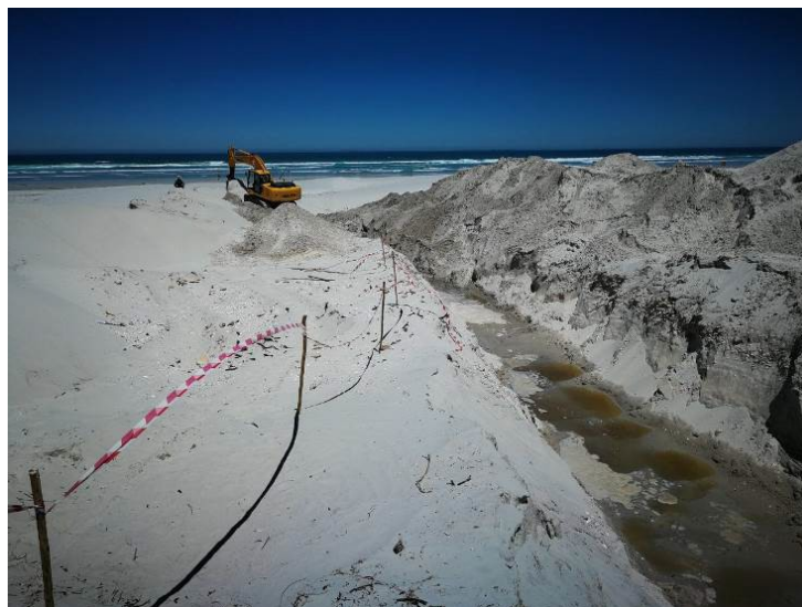
Figure 7 Example of excavations across the beach to bury the submarine cable
