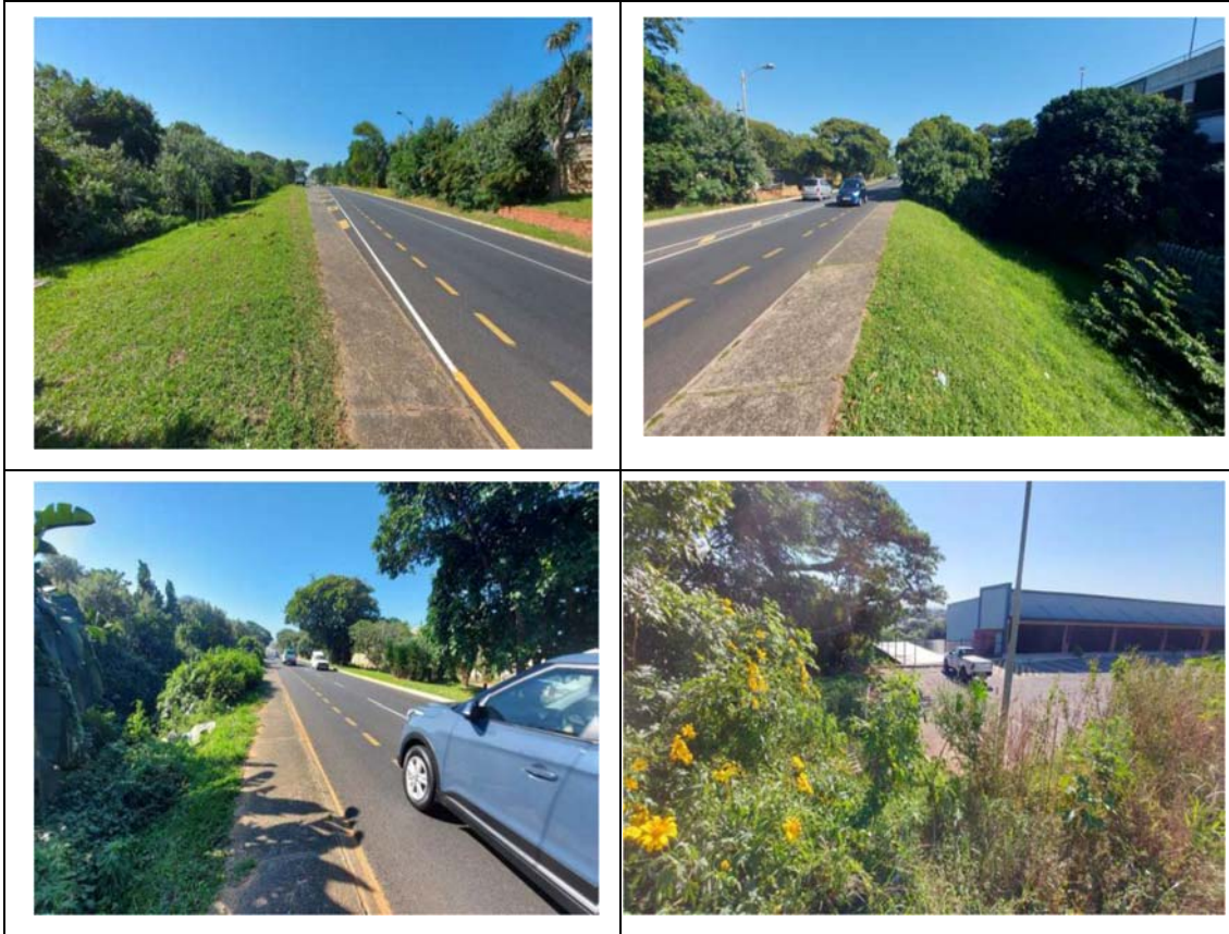
Plate 20 Photos showing grassed verges and coastal thicket along the terrestrial cable alignment between the Beach Manhole and Cable Landing Station at Amanzimtoti (Source: ENVASS, 2021)
