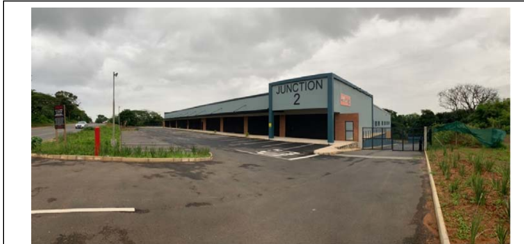
Plate 12 WIOCC's Cable Landing Station building at Umbogintwini
