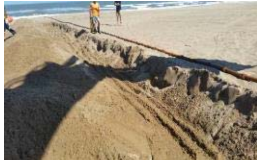
Plate 7 Landing of the cable on shore. Similar works will be undertaken for the landing of the 2AFRICA/GERA (East) Cable System
