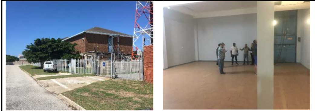
Plate 12 Telkom Exchange Building (left) and existing room inside the building (right) proposed to house the instrumentation for the 2AFRICA/GERA (East) Submarine Cable System (Gqeberha landing)
