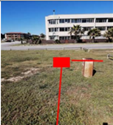
View of route towards Marine Drive, and Manhole position
