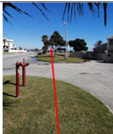
Trench across access road to Summerseas Beachfront Apartments
