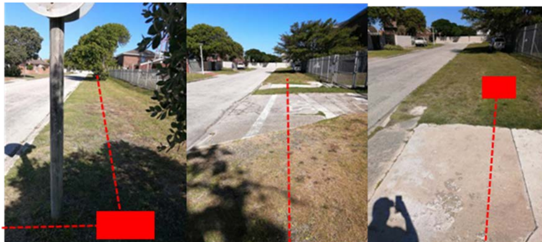
Install Manhole on outside of Summerstrand Telkom Exchange Building located to the right of the photographs
