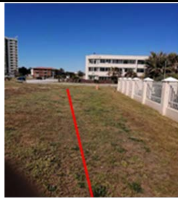
View of preferred route – Summerseas Beachfront Apartments fence visible to the right of the photograph.
