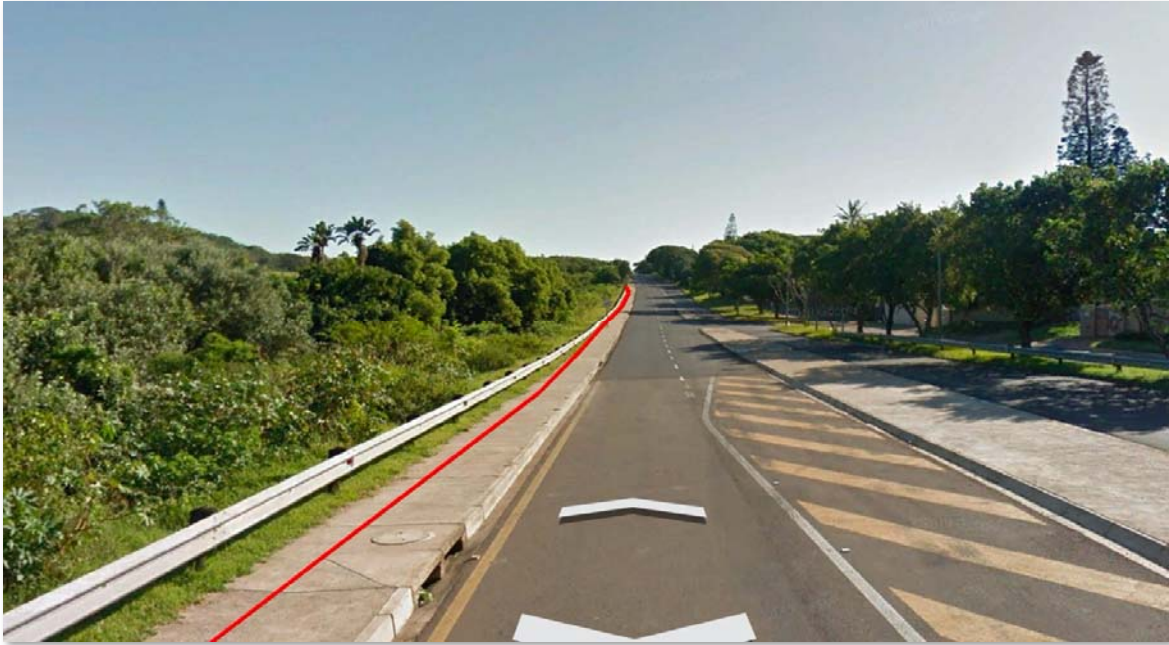
Plate 8: View along Kingsway showing routing of cable along existing pavement (Source: Google Earth).
