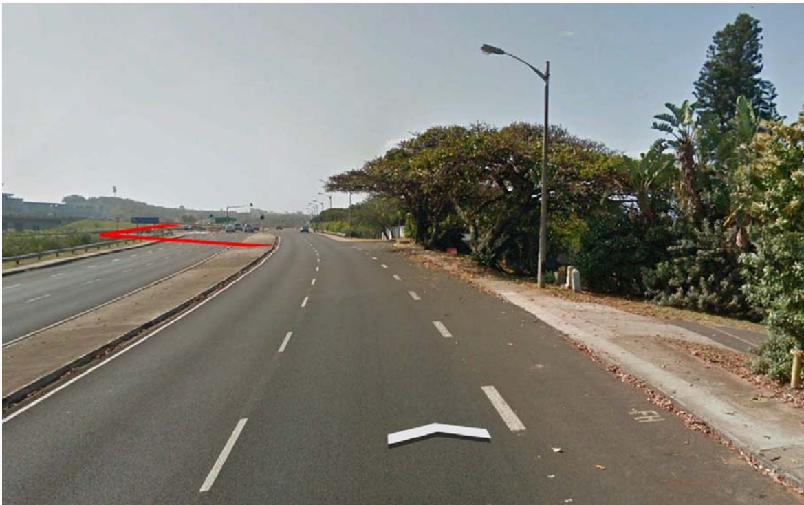
Plate 7: View north along Kingsway where cable crosses road (Source: Google Earth).
