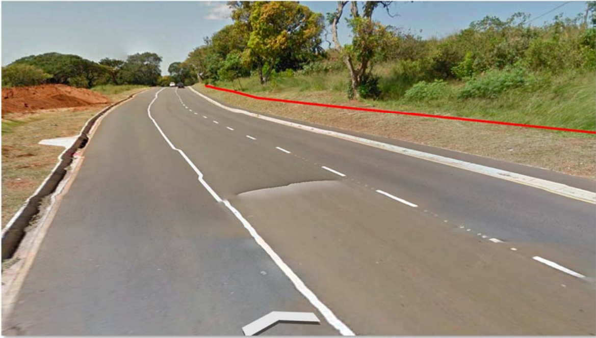
Plate 12: View of cable alignment along McGowan Place (Source: Google Earth).
