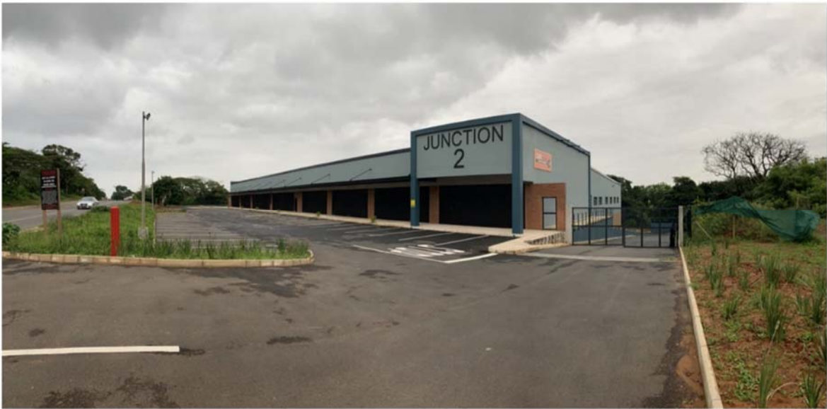
Plate 13: Cable Landing Station in McGowan Place (Source: ACER (Africa) Environmental Consultants 2021).
