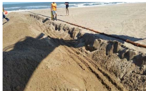
Plate 7 Landing of a cable on shore. Similar works will be undertaken for the landing of the 2AFRICA (West) Cable System (Yzerfontein landing)
