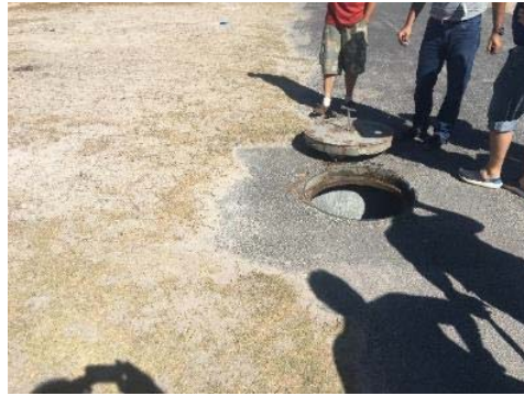
Manhole along the WACS front haul alignment
