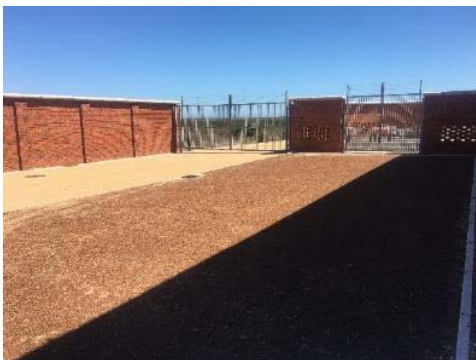
Area at the WACS CLS which is available for extending the CLS to accommodate the 2AFRICA cable
