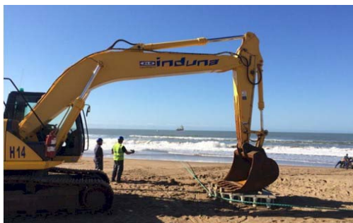
Plate 7 Landing of a cable on shore. Similar works will be undertaken for the landing of the 2AFRICA (West) Cable System (Yzerfontein landing)
