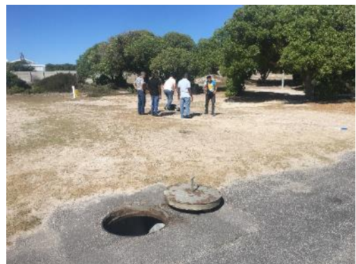
Existing WACS man hole on the front haul alignment
