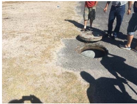
Manhole along the WACS front haul alignment
