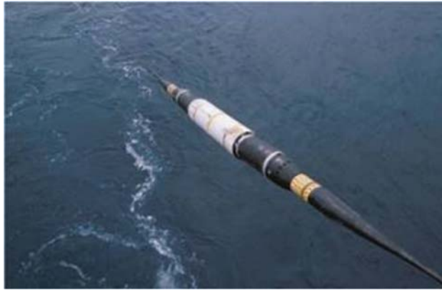
Plate 3 Example of a repeater
