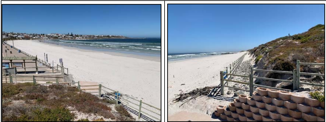
Plate 16 No vegetation is present along the proposed cable route alignment at Yzerfontein Beach, where the foredune is transformed by a seawall for erosion control (left photo). The vegetated dune cordon further north will not be affected (right photo)
