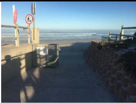
Beach access path adjacent to the existing WACS pipe conduit to the beach
