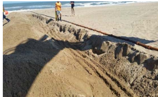
Plate 7 Landing of a cable on shore. Similar works will be undertaken for the landing of the 2AFRICA (West) Cable System (Yzerfontein landing)
