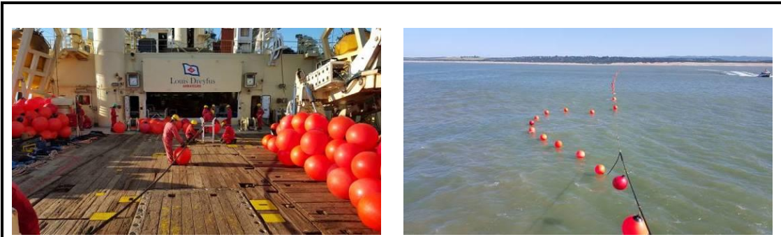
Plate 8 Bringing the cable to shore from the cable laying vessel. Cable is buoyed off and pulled to shore with smaller vessels.
