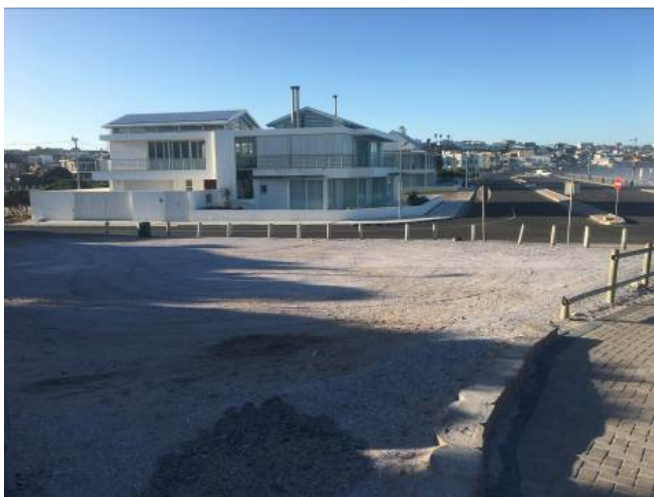
Figure 7 Location of the WACS BMH at Yzerfontein Main Beach
