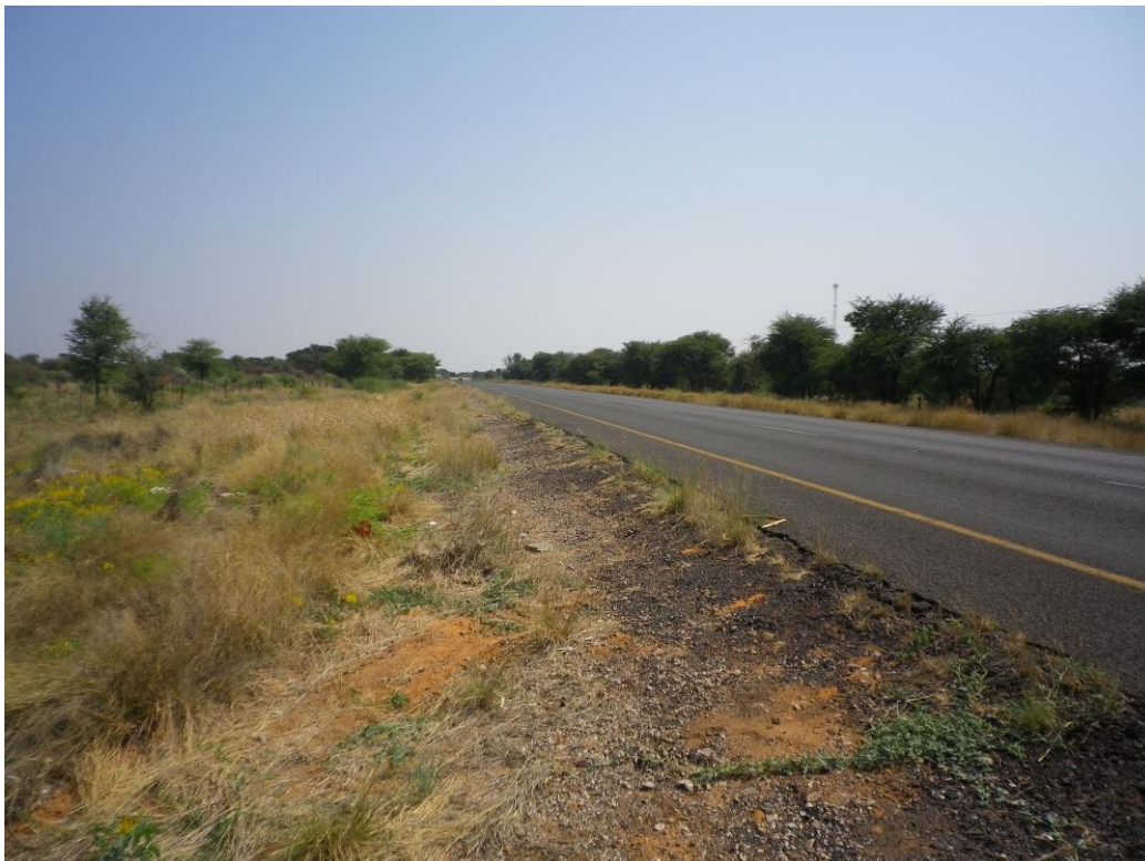
Photo F: View of where proposed powerline will cross the R380 road.
