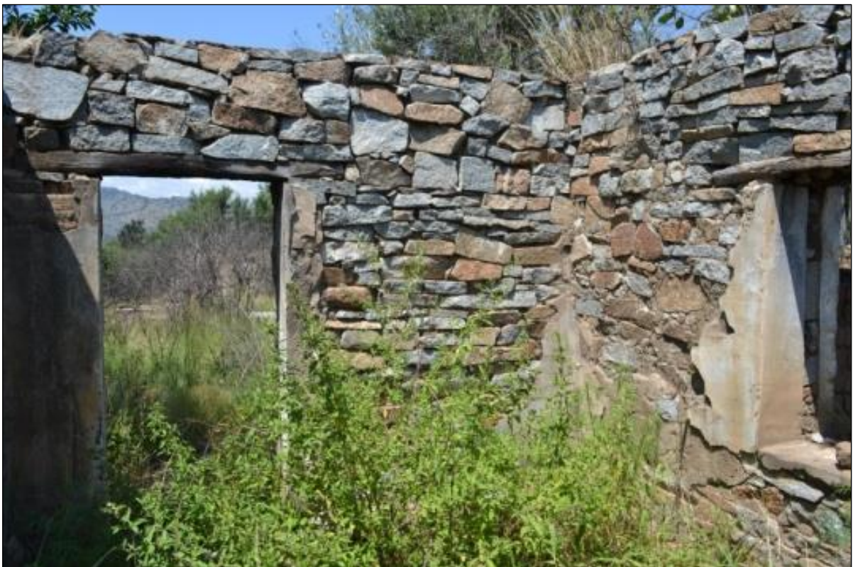
Figure 76 – Interior view of a section of the historic farm dwelling at feature DBAP 15A. Photograph was taken in 2015 by Mauritz Naudé.
