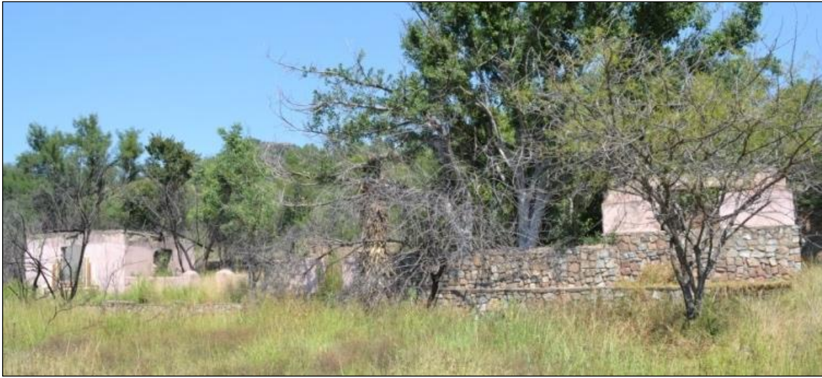
Figure 79 – General view of the building at feature DBAP 15C. Photograph was taken in 2015 by Mauritz Naudé.
