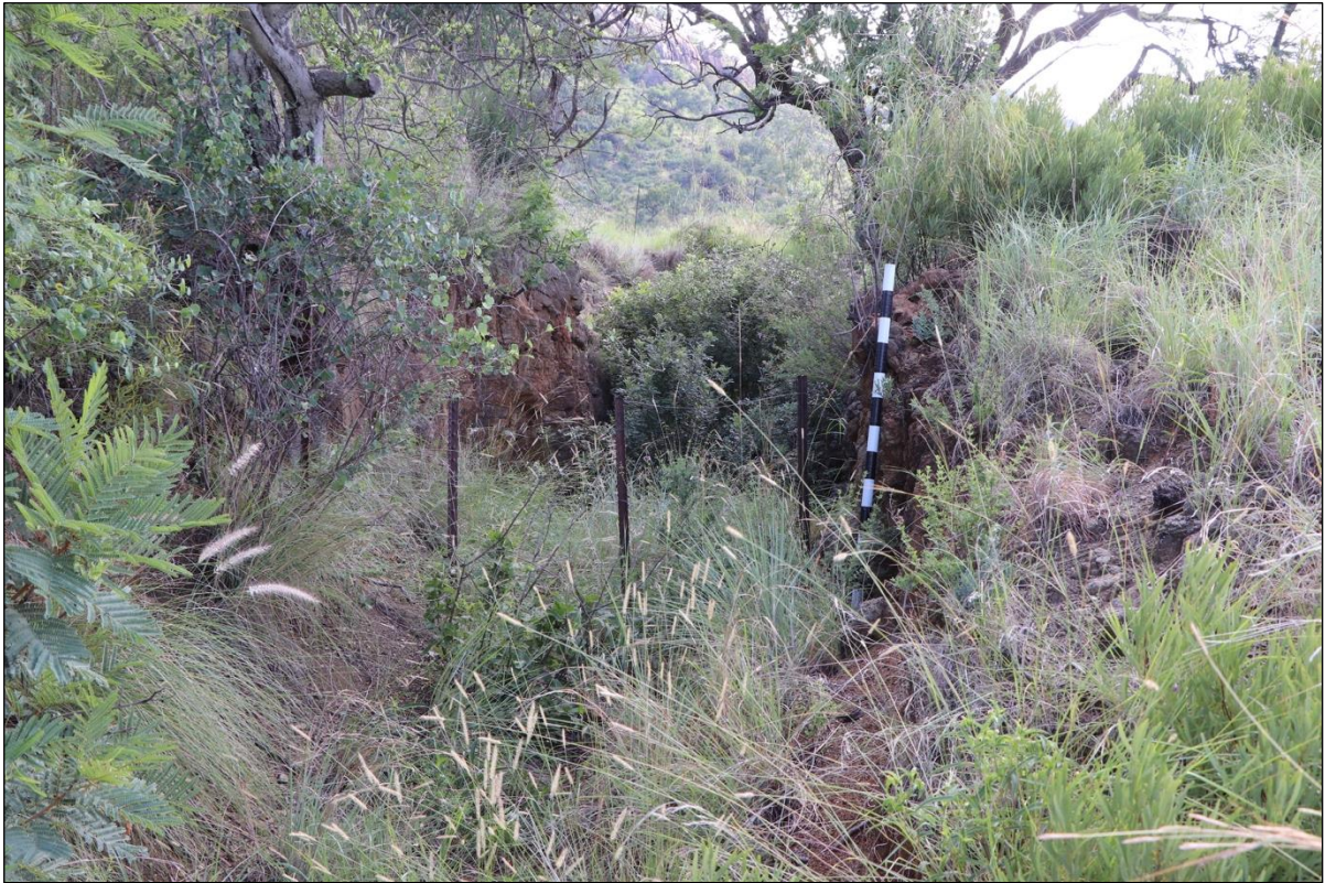
Figure 70 – The entrance of the adit at site DBAP 12. Scale in 10cm increments.
