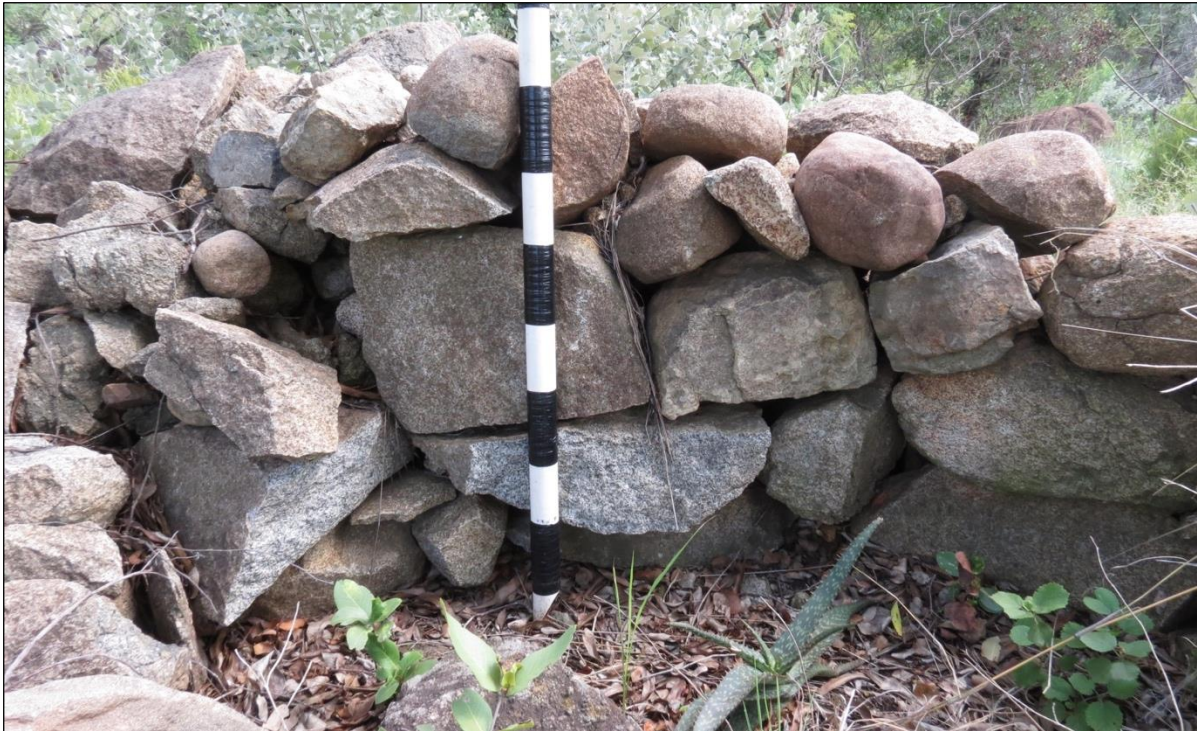
Figure 55 – Side view of a section of the enclosure wall at DBAP 9B. Scale in 10cm increments.
