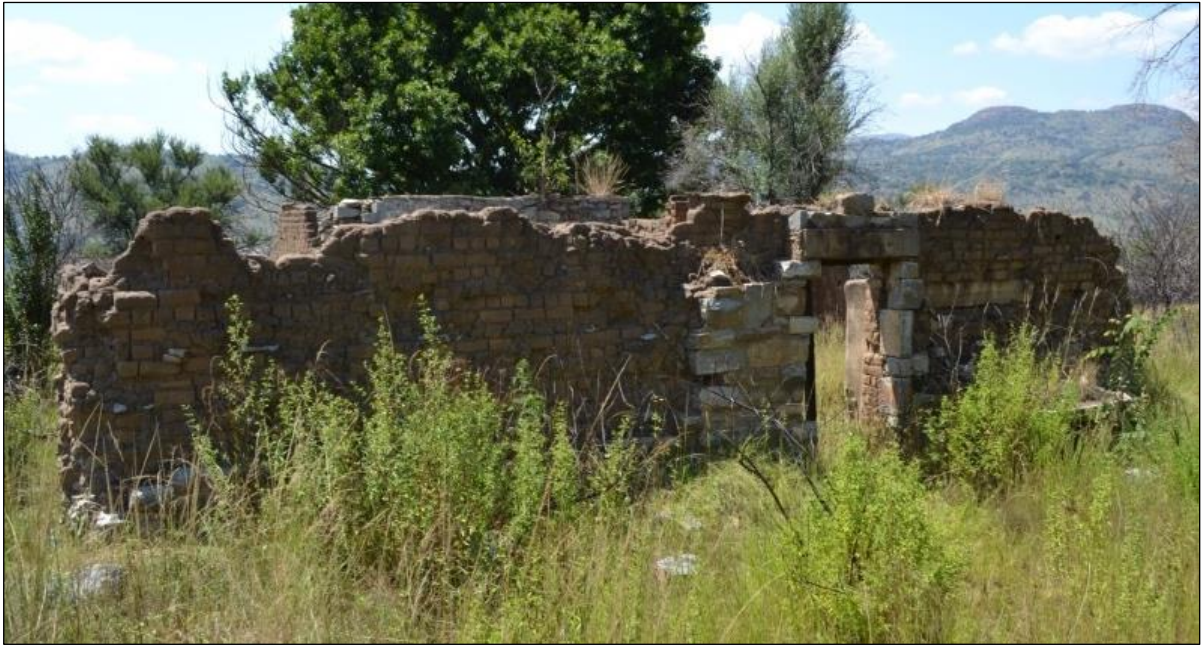
Figure 75 – General view of historic farm dwelling at feature DBAP 15A. Photograph was taken in 2015 by Mauritz Naudé.
