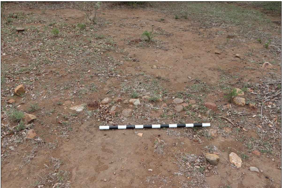
Figure 108 – A section of low terrace walling from site DBAP 26 can be seen in this photograph. The scale is in 10cm increments.
