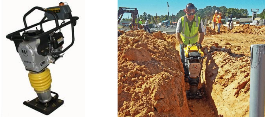
Figure 3: Example of trench backfilling and compaction.
