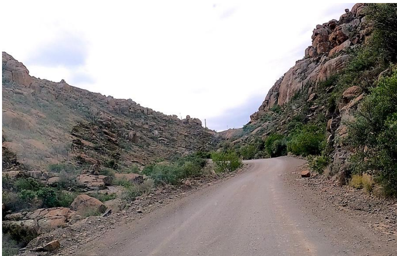
Figure 29: Picturesque Molteno pass R381 route winding between dolerite formations. Powerline pylons visible on the far skyline.
