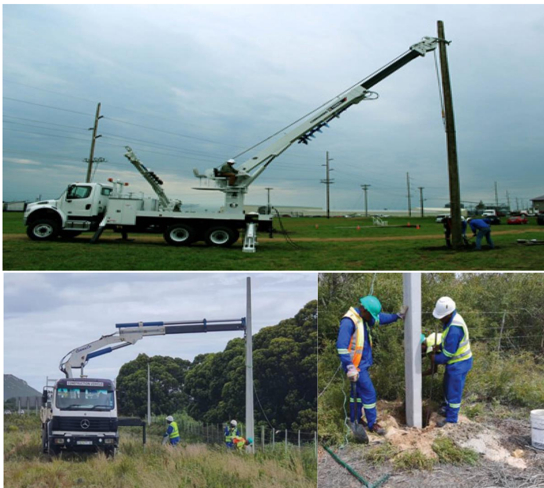
Figure 8: Example of a truck used to plant timber (top) and concrete (bottom) poles.
