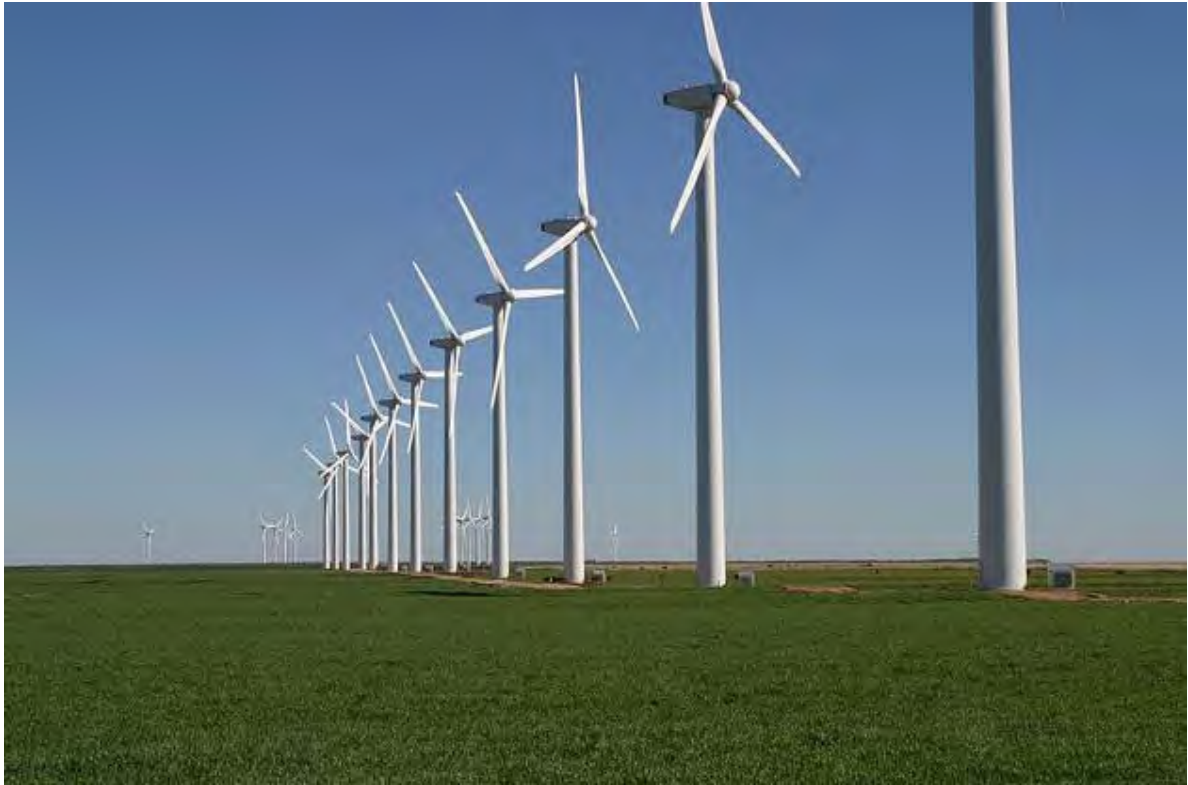
Figure 3.1: Brazos Wind Ranch located in Texas, USA 16
