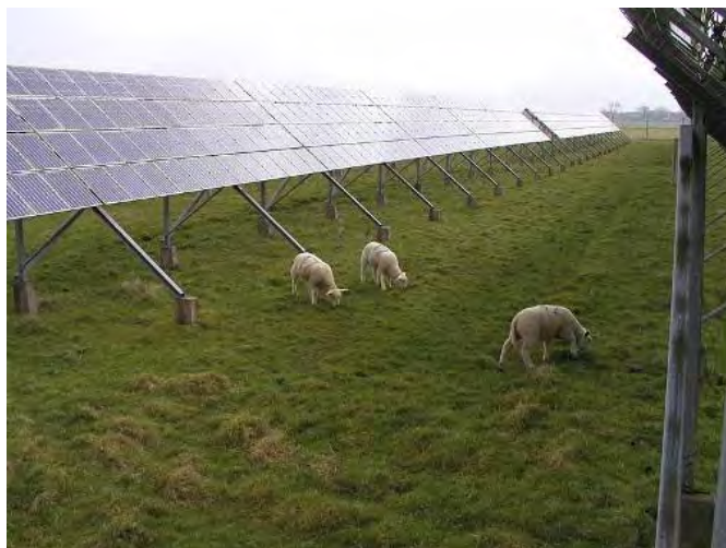
Figure 3.10: PV ground mounted system 21
