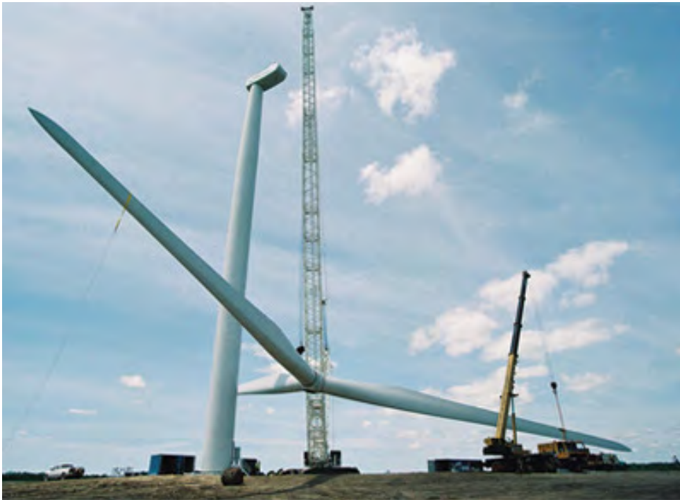
Figure 3.3: A wind turbine in the process of being erected 18
