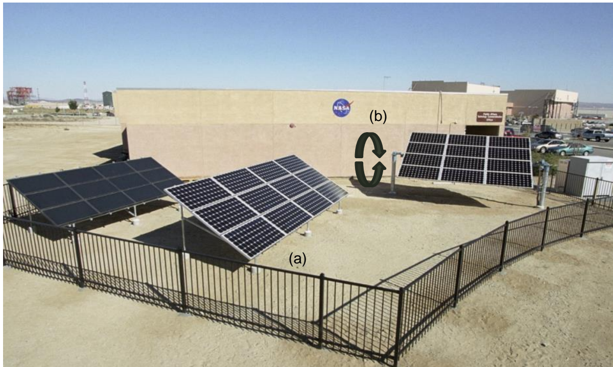
Figure 3-14 Fixed axis tracking system (a) and single axis tracking system (b) (courtesy Mulilo)
