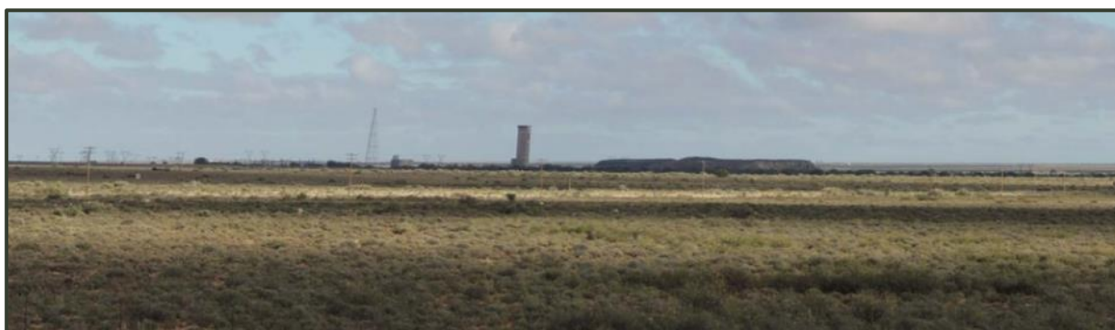
Figure 5-12 View of existing mining infrastructure of Copperton Mine (VRM, 2013)
