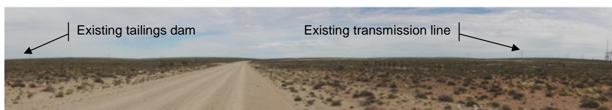
Figure 5-14 Area visible to community: R357 westbound where the proposed panels would be visible on either side of the road (VRM, 2013)
