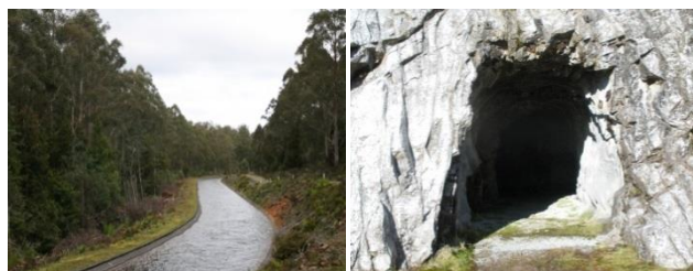
Figure 5 | Water conveyance alternatives- open canal vs. tunnel
