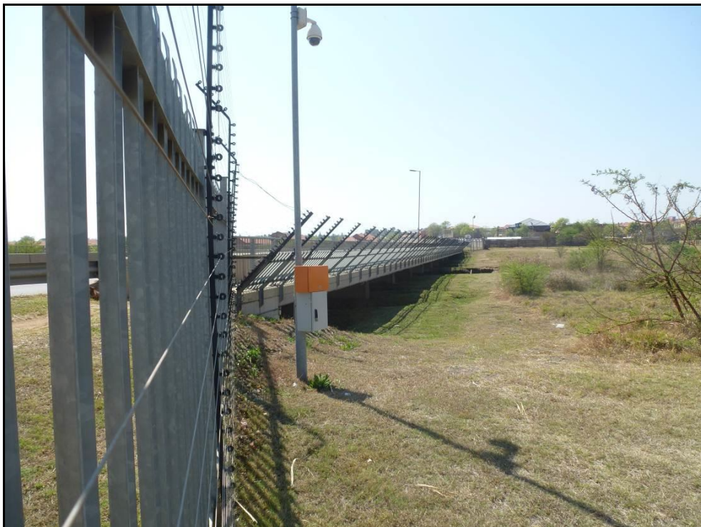
Figure 18. Photo of an existing bridge along Bougainvillea Drive to the south of the site. The proposed Tsamma Road Bridge will be very similar to this bridge.
