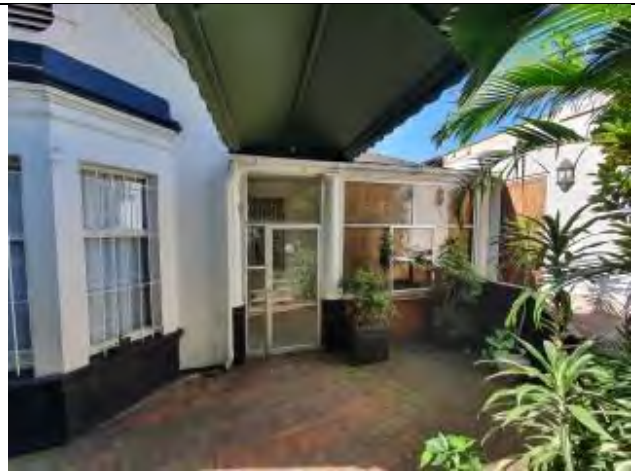
Figure 1.8: Enclose veranda at front entrance
