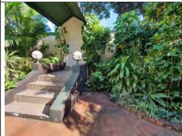
Figure 1.9: Existing stairs to street level
