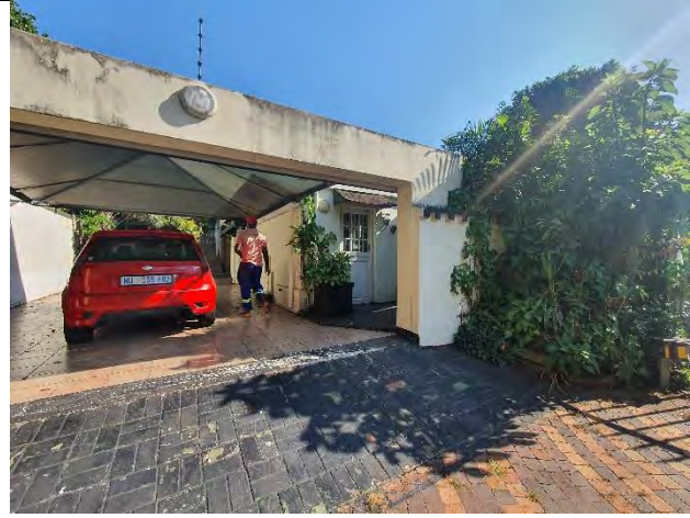
Figure 1.12: Rear vehicle entrance from access lane off Botanic Lane
