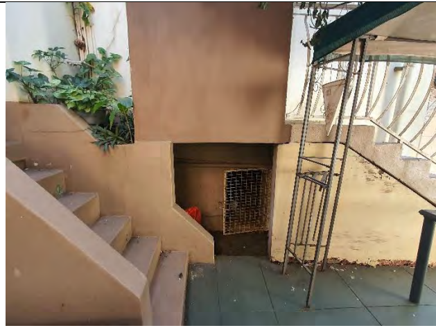
Figure 1.14: Stairs from parking area to the original house
