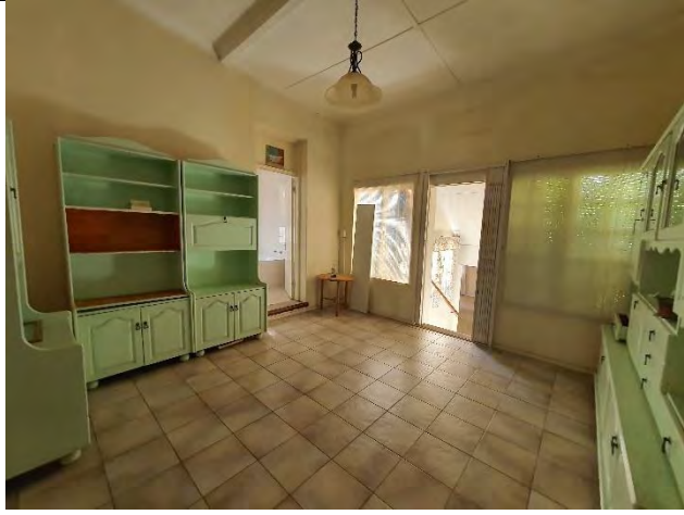
Figure 23: Rear of existing original dwelling and entrance to the new extension at lower level
