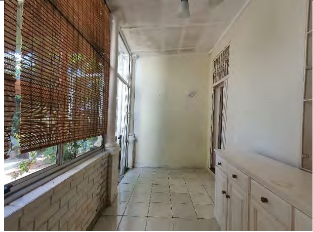
Figure 20: Existing enclosed veranda on original portion of the house
