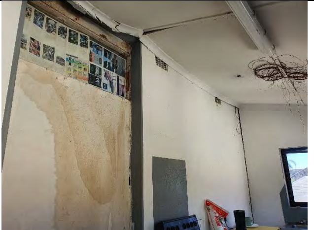
Figure 3.16: Condition of existing ceilings & drywalls
