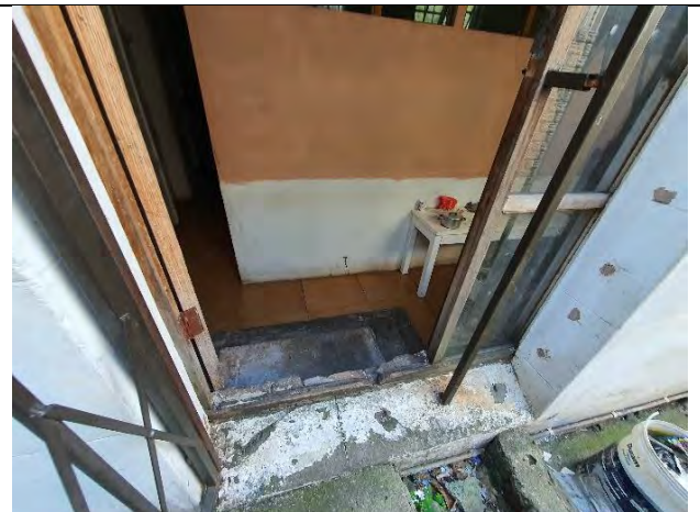
Figure: 3.4: Entrance to lower ground floor
