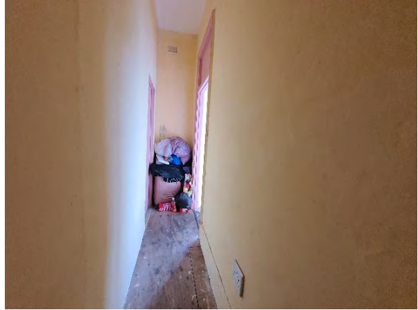
Figure 2.14: Existing entrance passage
