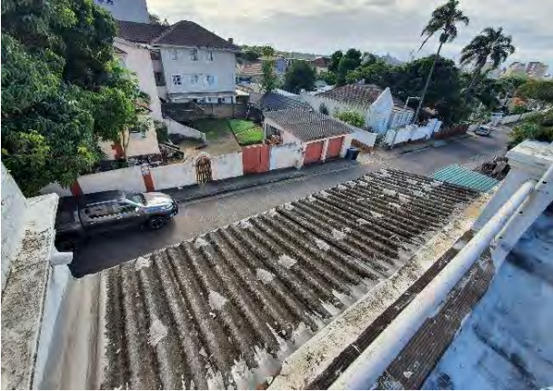
Figure 1.13: View from the roof looking NE
