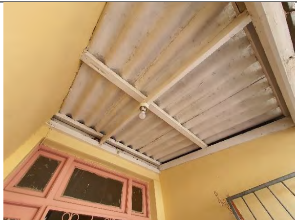
Figure 2.12: Existing asbestos roofing over entrance
