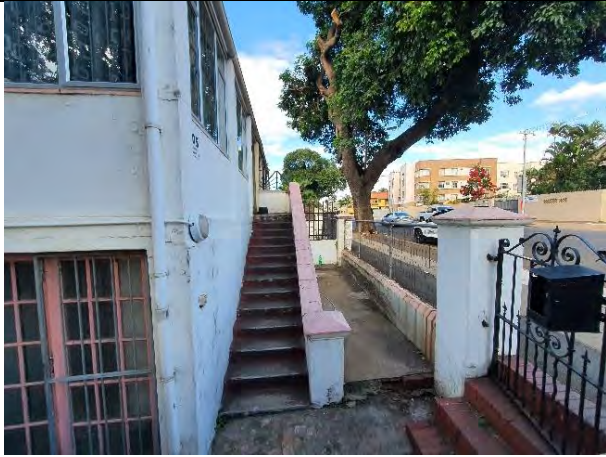
Figure 2.1: Entrance stair below street level
