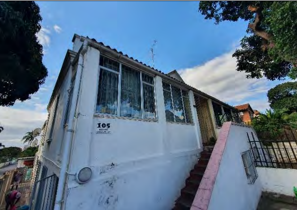
Figure 1.16: Access to 105 from the NW corner of the site at corner of Botanic Gardens Rd & Botanic Ave
