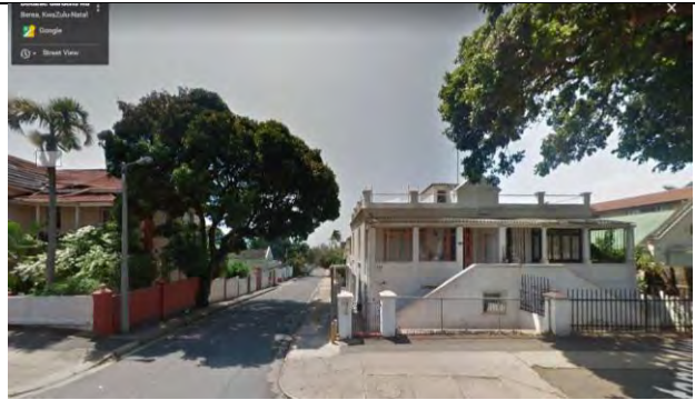
Figure 1.5: Street view looking SE down Botanic Ave
