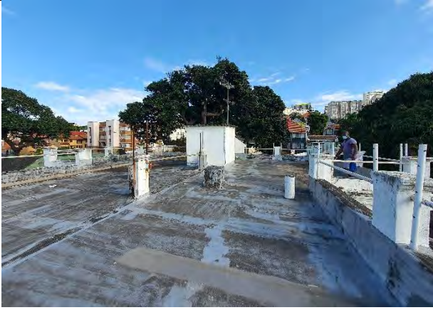
Figure 1.11: View of roof slab over 105 & 101
