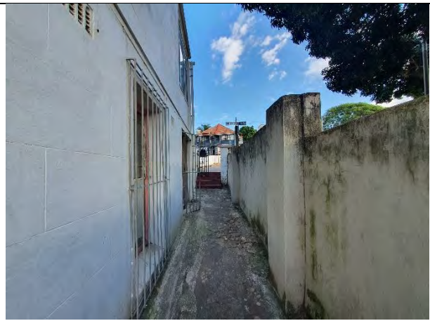
Figure 2.4: Side yard parallel to Botanic Avenue
