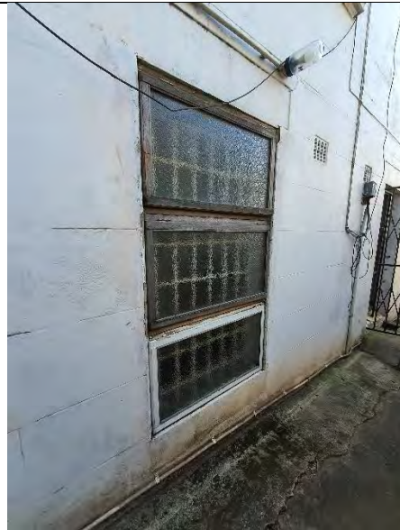
Figure 3.18: External lower ground floor windows
