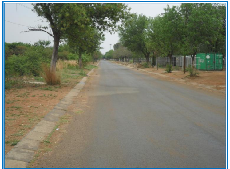
Plate 23: View of Scott Street (direction south)
