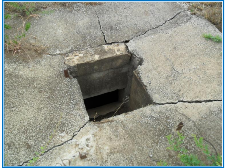
Plate 8: View of existing stormwater inlets
