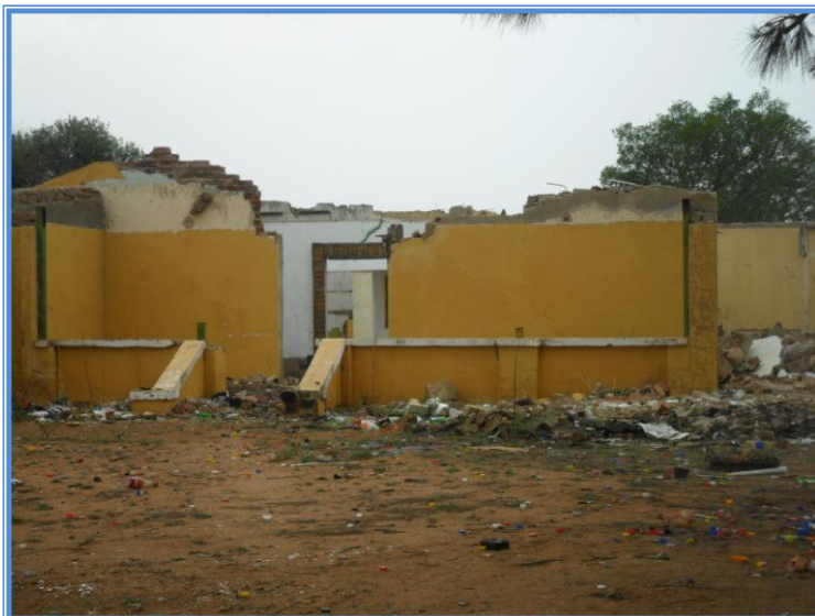
Plate 1: Demolished dwelling house (Holding 19)
