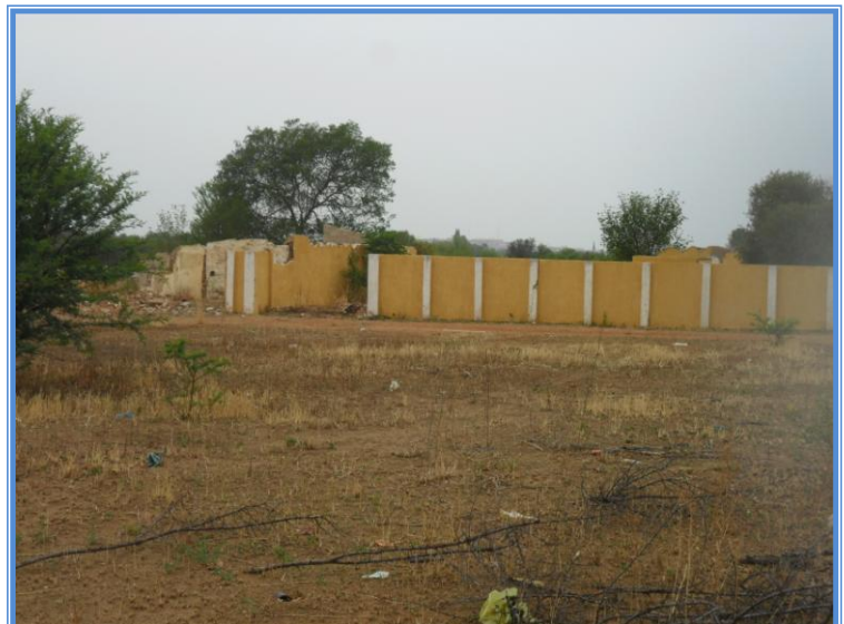
Plate 2: Demolished dwelling house (Holding 19)
