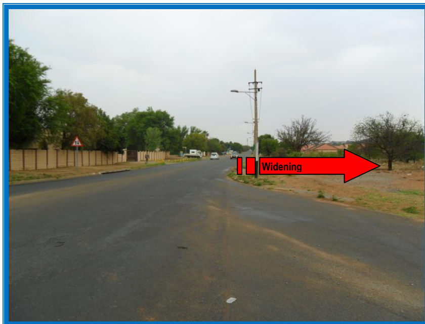
Plate 24: View of the section of Ian Street proposed for widening
