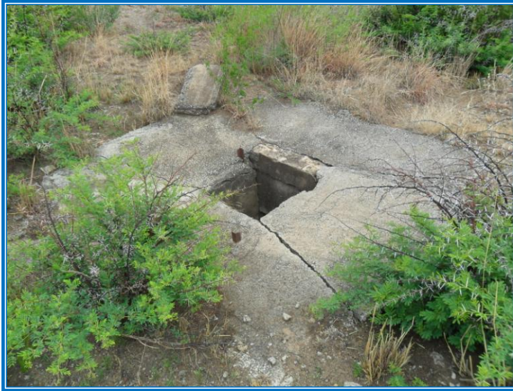
Plate 7: View of existing stormwater inlets
