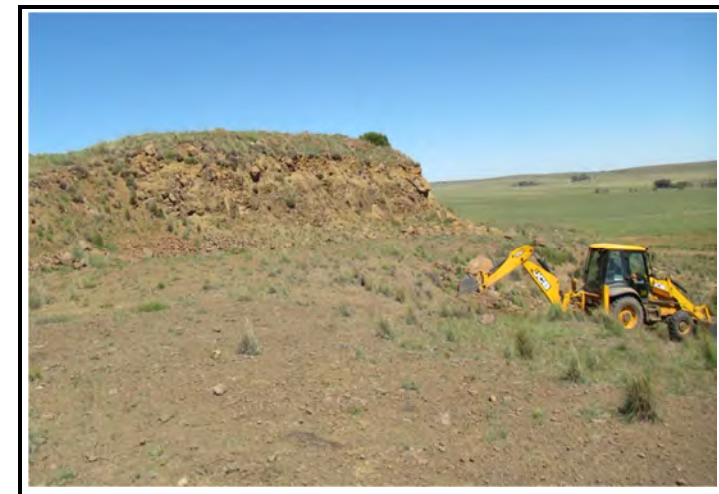
View of potential borrow pit target area - note existing borrows
