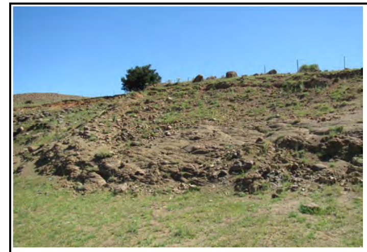
View of existing borrow pit excavation showing deep weathering
