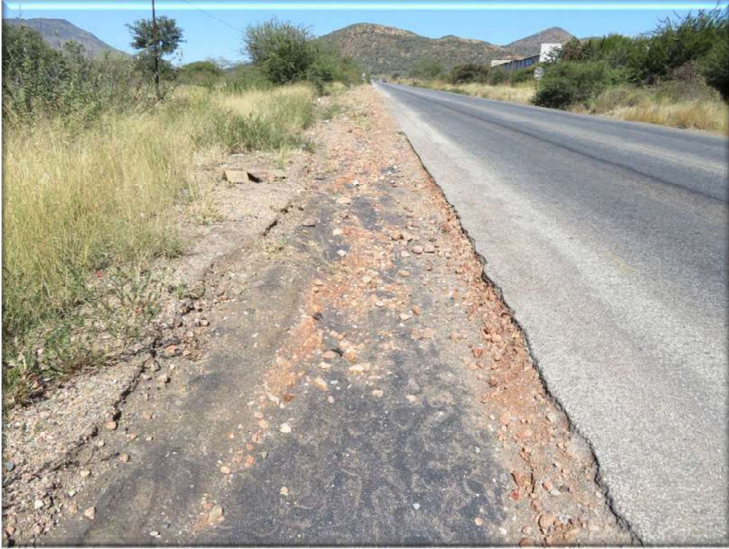
Figure 6-2 Road drainage adjacent to Site 1
