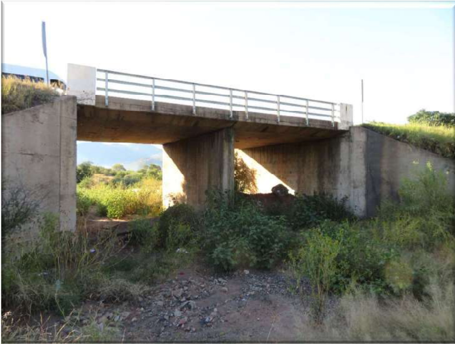
Figure 6-8 R555 bridge over first and major channel through Site 5
