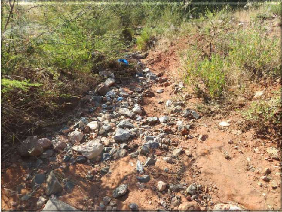
Figure 6-11 Third drainage channel on Site 5 (looking downstream)
