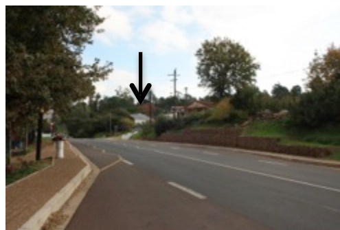
Figure 8 View south from the R310 scenic route with the existing house on the site visible in the centre of photo (white wall and grey roof, arrow).
