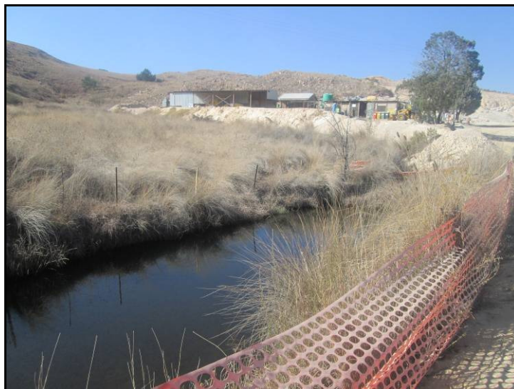
Photo 3.12: Small dam in drainage area
