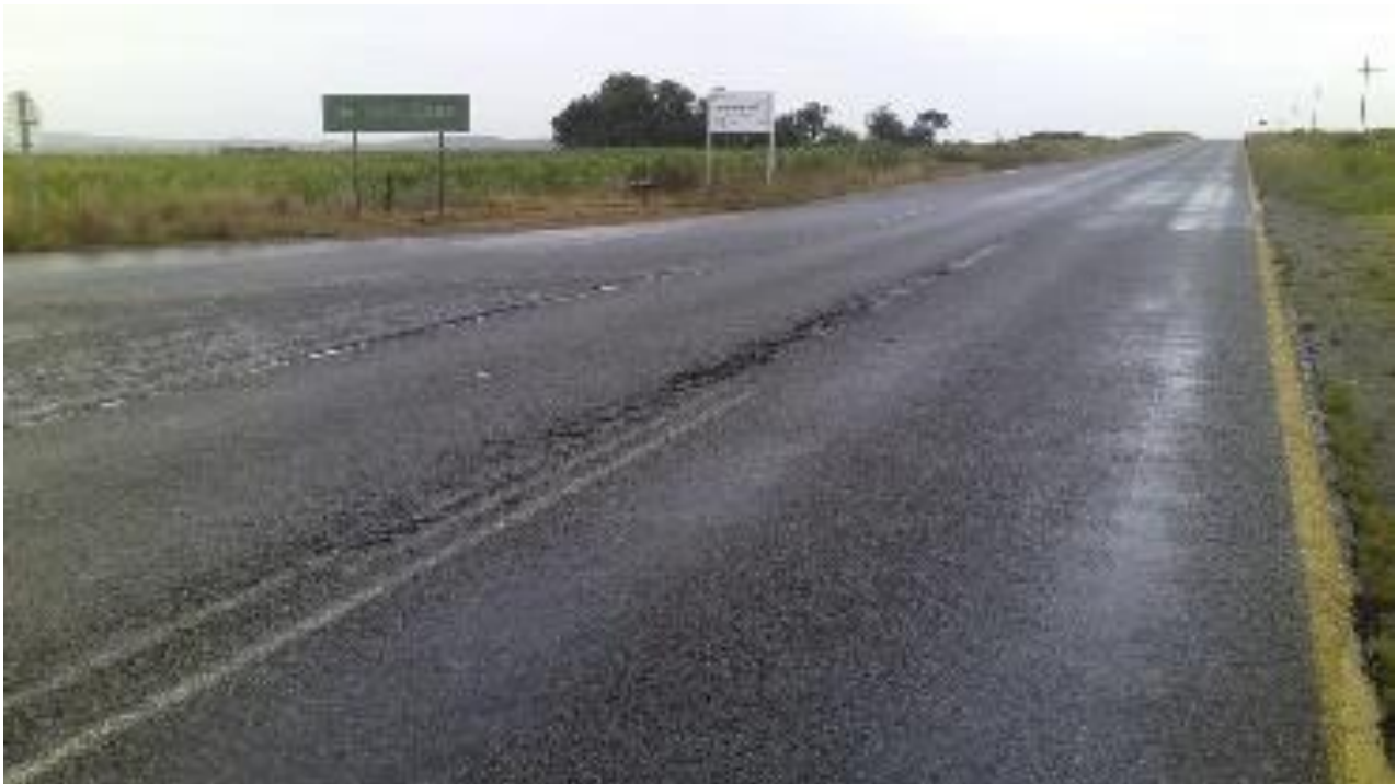
Figure 7-15: A view of the Boundary Road. The road links the R42 and R59 roads within the surrounding area.
