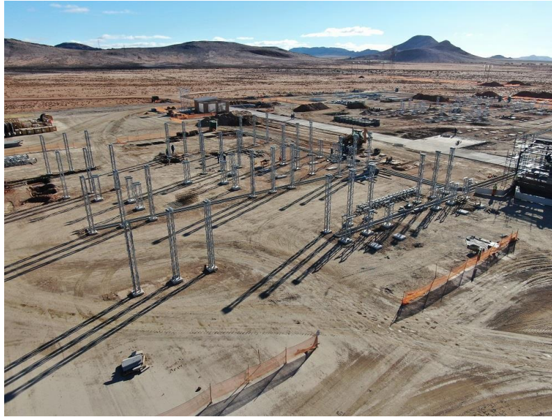
Figure 5-3: A Switching Station under construction 20 .
