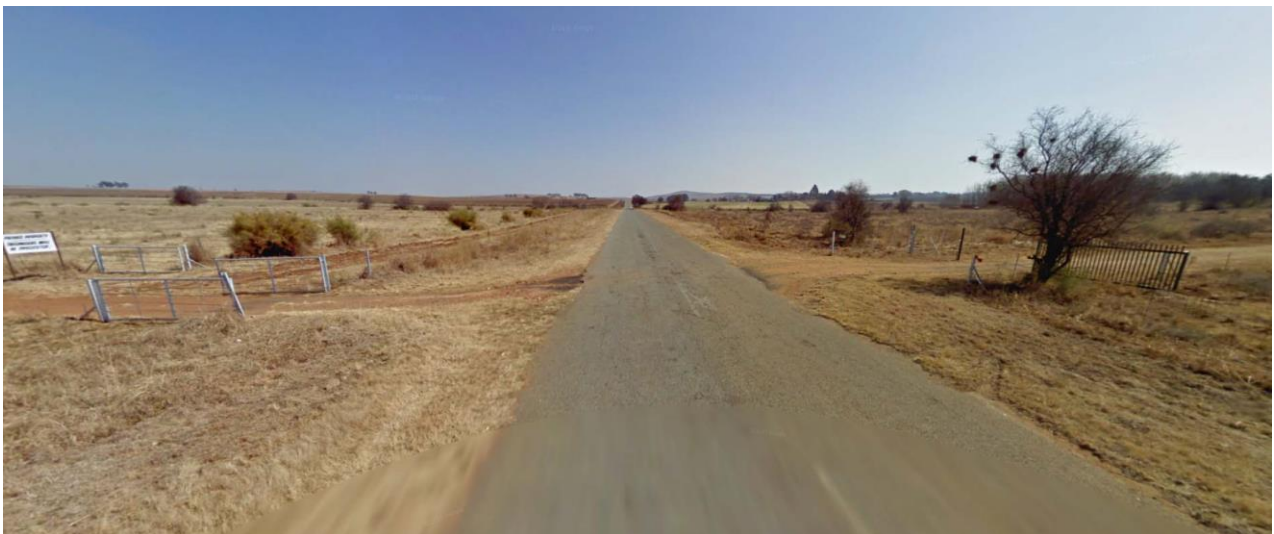
Figure 7-16: A view of the Road S 171. The road will provide direct access to the project site of the proposed project.
