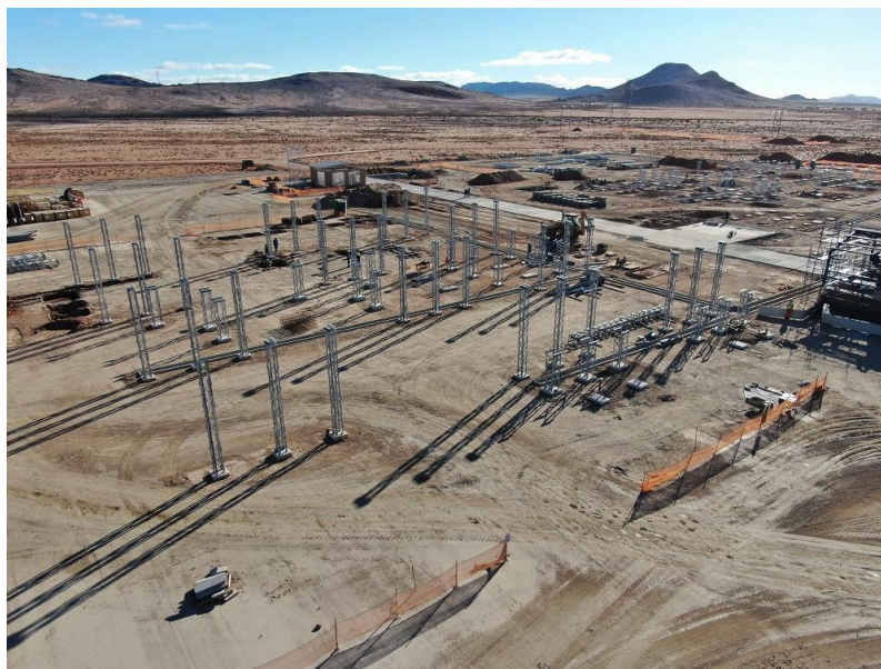
Figure 5-3: A Switching Station under construction 20 .
