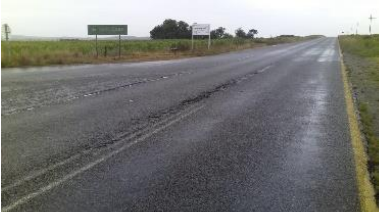
Figure 7-15: A view of the Boundary Road. The road links the R42 and R59 roads within the surrounding area.
